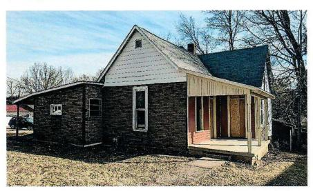
This is the Smith Avenue view, showing the front of the house and some aluminum siding removed. The rest of the aluminum siding and the insulbrick will be removed. The existing wood siding will be repaired (or replaced if necessary) and painted to match the porch, which was opened up, repaired and painted by BRI just before we bought the house.
