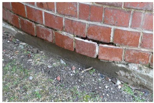
Photo 7 Spalling extends to the base of the stack.
