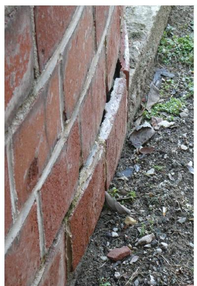
Photo 8 The face shells are splitting off from the body of the brick.
