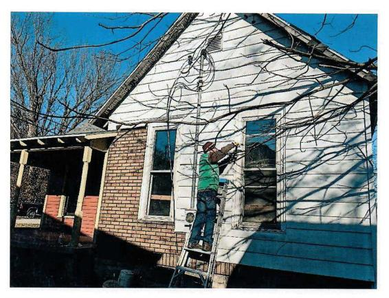
The west side of the house. The aluminum and insulrick siding will be removed and the clapboards repaired or replaced before painting.
