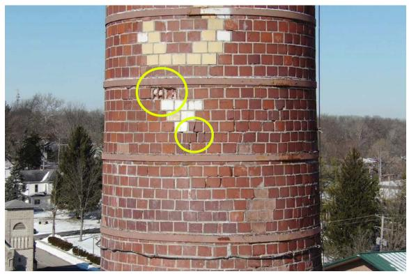
Photo 5 New spalls are highlighted in this 2022 photo.
