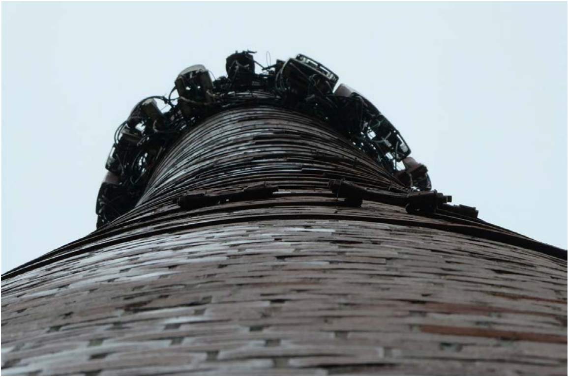
Photo 1 Looking up the wall of the stack on the southeast face.
