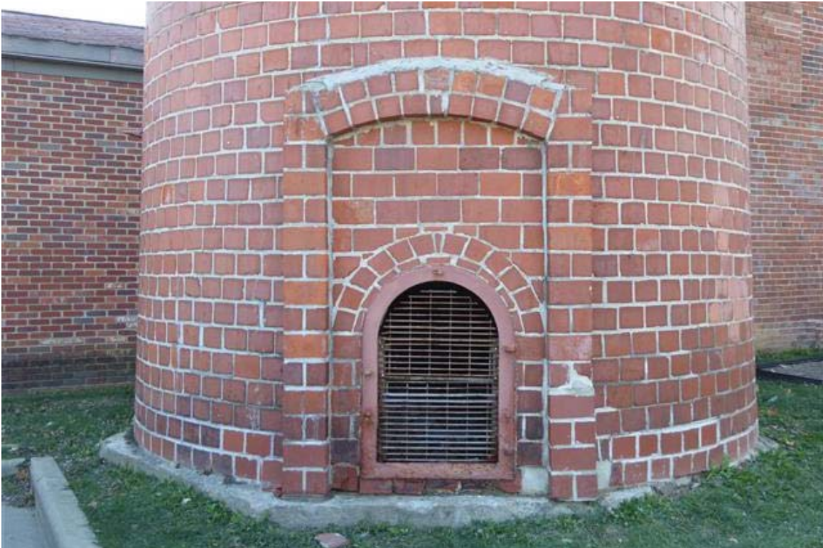
Photo 13 Opening at the base of the stack.
