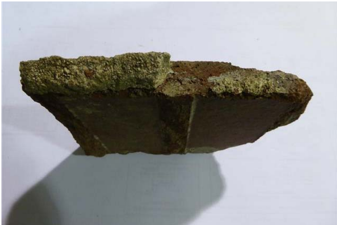
Photo 18 The outer face shell is only 3/4 inches thick.
