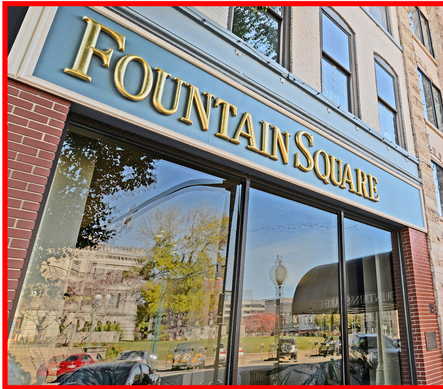
Existing Sign Board, Size 244”w x 34”h Existing Materials Include painted formed plastic letters that are stud mounted.
