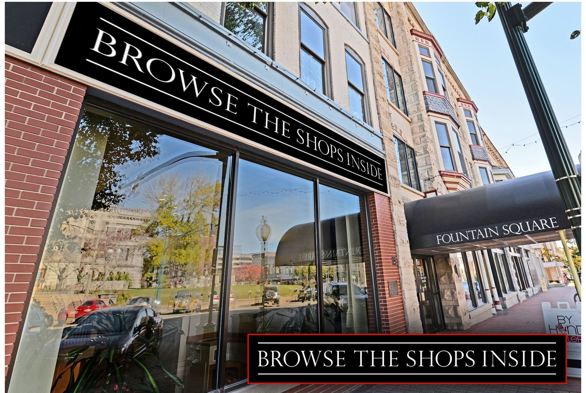
Updated Sign Mockup proposes to use the existing signage structure. New dimensional letters (172”w x 24”h) will be stud mounted. The lettering will either be the same type of formed plastic or acrylic. Any holes will be patched, and the board will be painted. The sign will also include two raised elongated bars.
