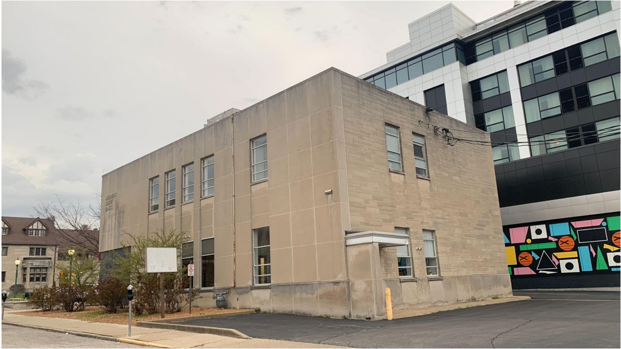
Figure 6: Facades facing Washington Street and the parking lot
