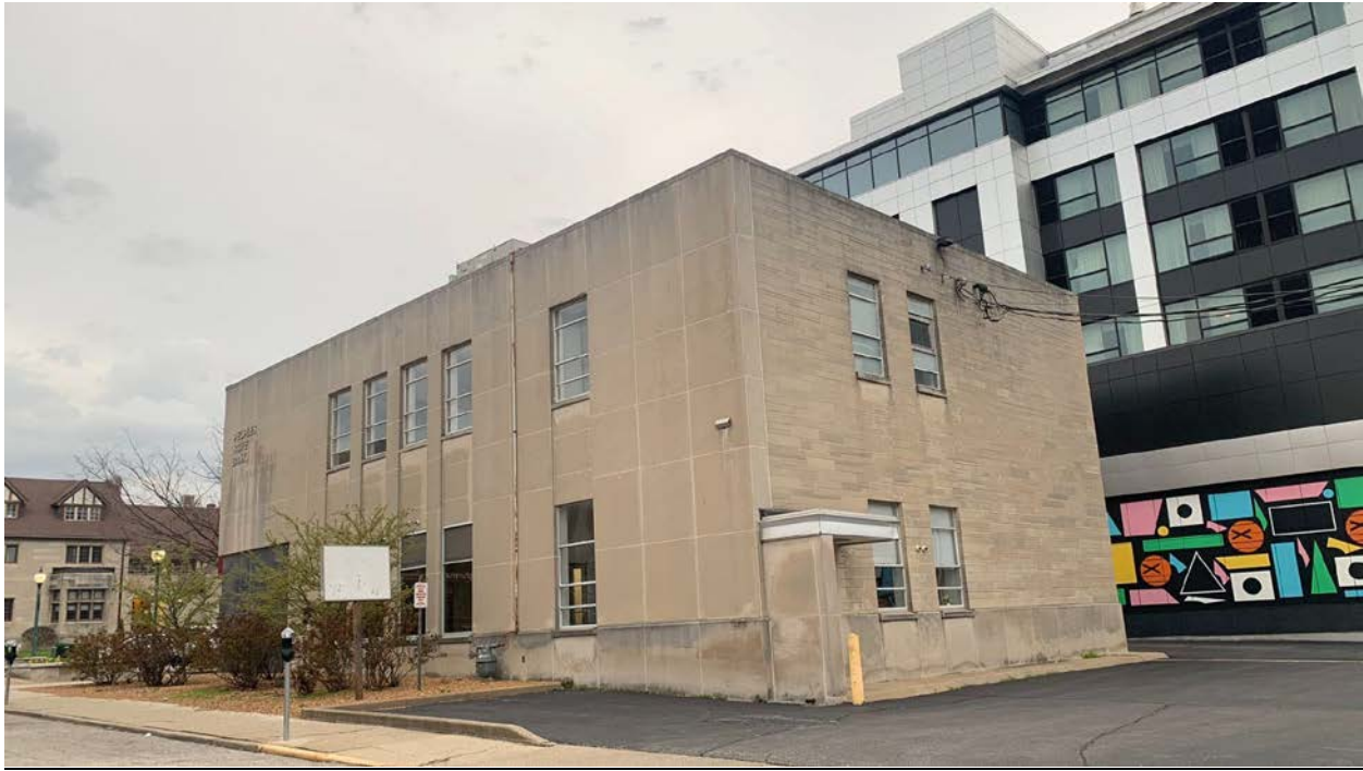
Figure 6: Facades facing Washington Street and the parking lot
