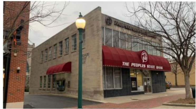
Figure 5: Facade facing Kirkwood Avenue and the drive through
