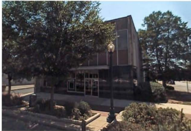
Figure 4: Google Street View Image from 2007 with the original metal canopy intact
