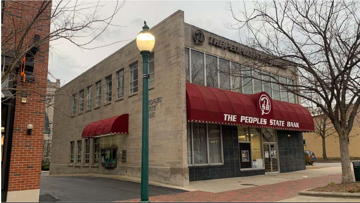
Figure 5: Facade facing Kirkwood Avenue and the drive through
