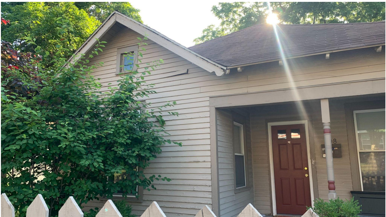
Image 12: West facade with the front entrance of the parsonage, bungalow, 2022 (photo by staff)
