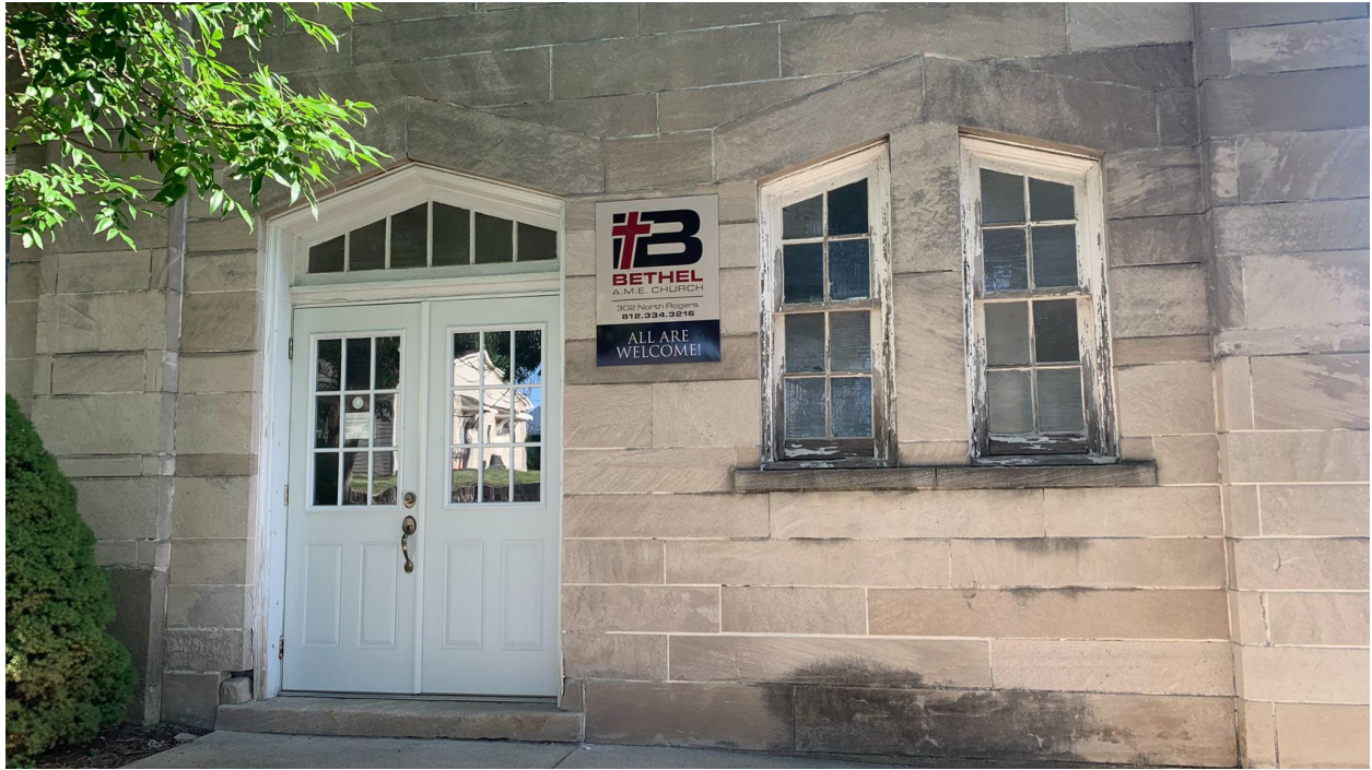
Image 9: Original windows facing southward, 2022 (photo by staff)
