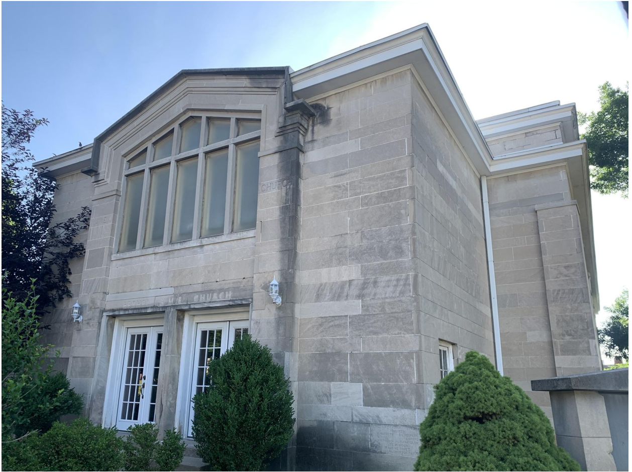
Image 6: Front of the church structure facing west, 2022 (photo by staff)
