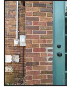
D EXIST. CONDITIONS PHOTO NTS
