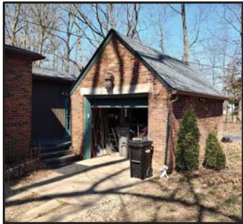
K EXIST. CONDITIONS PHOTO NTS
