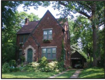
A EXIST. CONDITIONS PHOTO NTS
