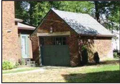
B EXIST. CONDITIONS PHOTO NTS
