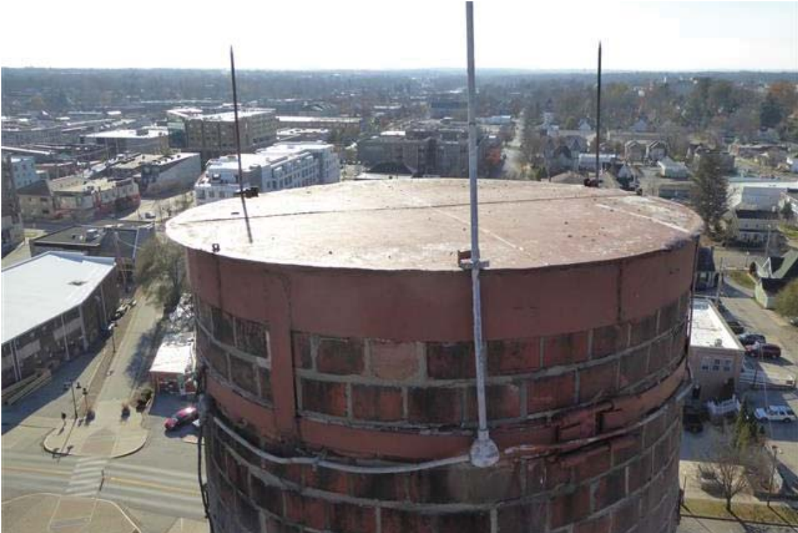
Photo 11 The top of the stack has been capped with a steel plate.
