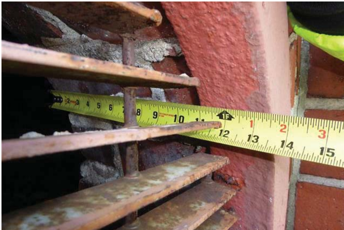
Photo 14 Wall thickness at the opening is 13 inches or 3 wythes of brick. This flares out to 5 wythes of brick or 20 inches in thickness on the sides of the opening.
