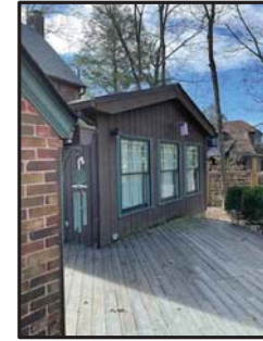
J EXIST. CONDITIONS PHOTO NTS
