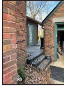
C EXIST. CONDITIONS PHOTO NTS
