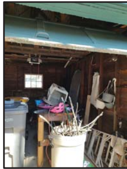
L EXIST. CONDITIONS PHOTO NTS
