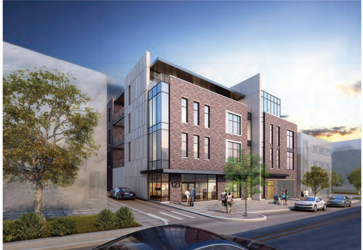
VIEW LOOKING NORTHEAST FROM KIRKWOOD
