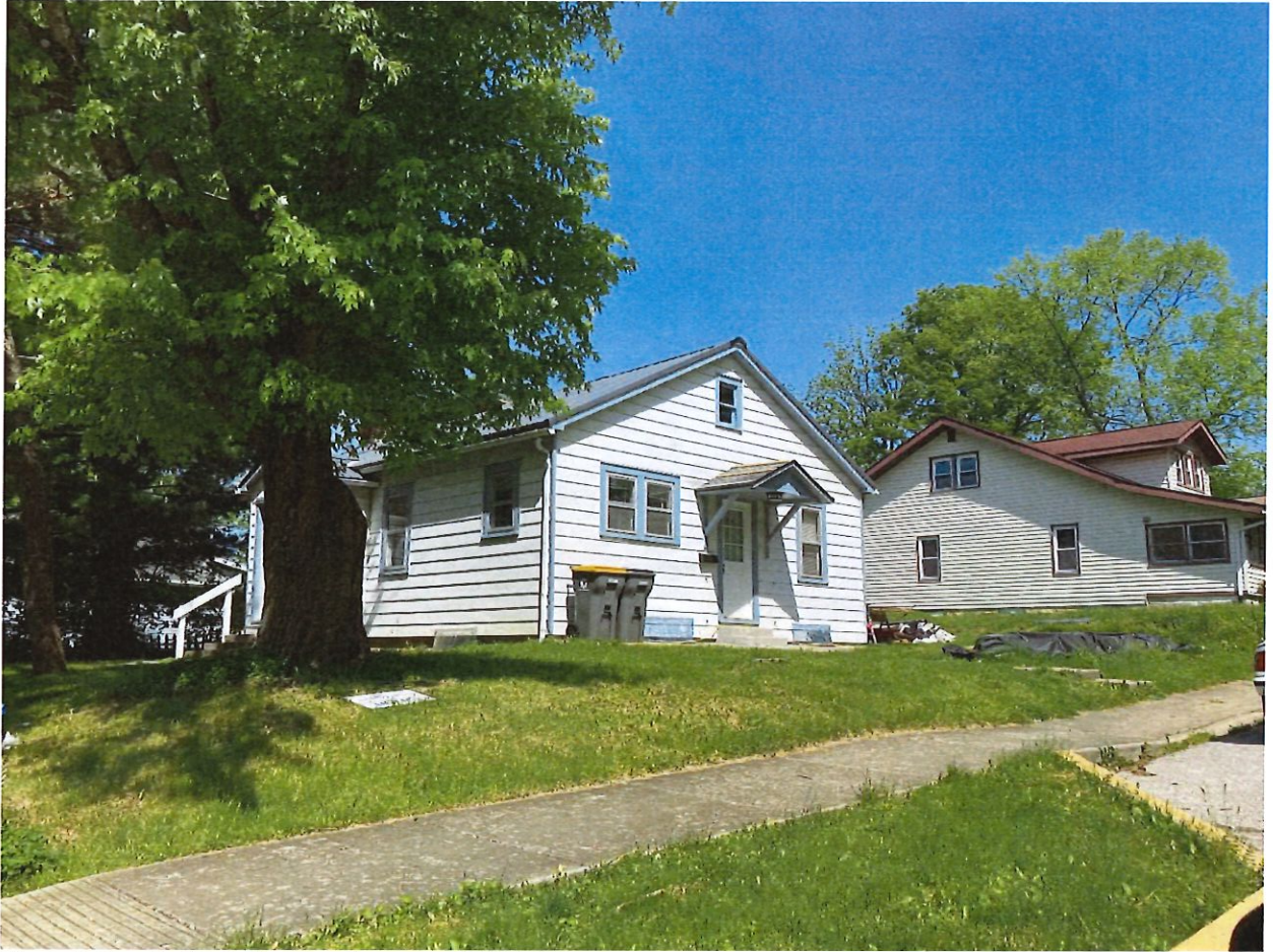
Photo 2: Roof of 221 E. Allen Street on 05/12/2022.
