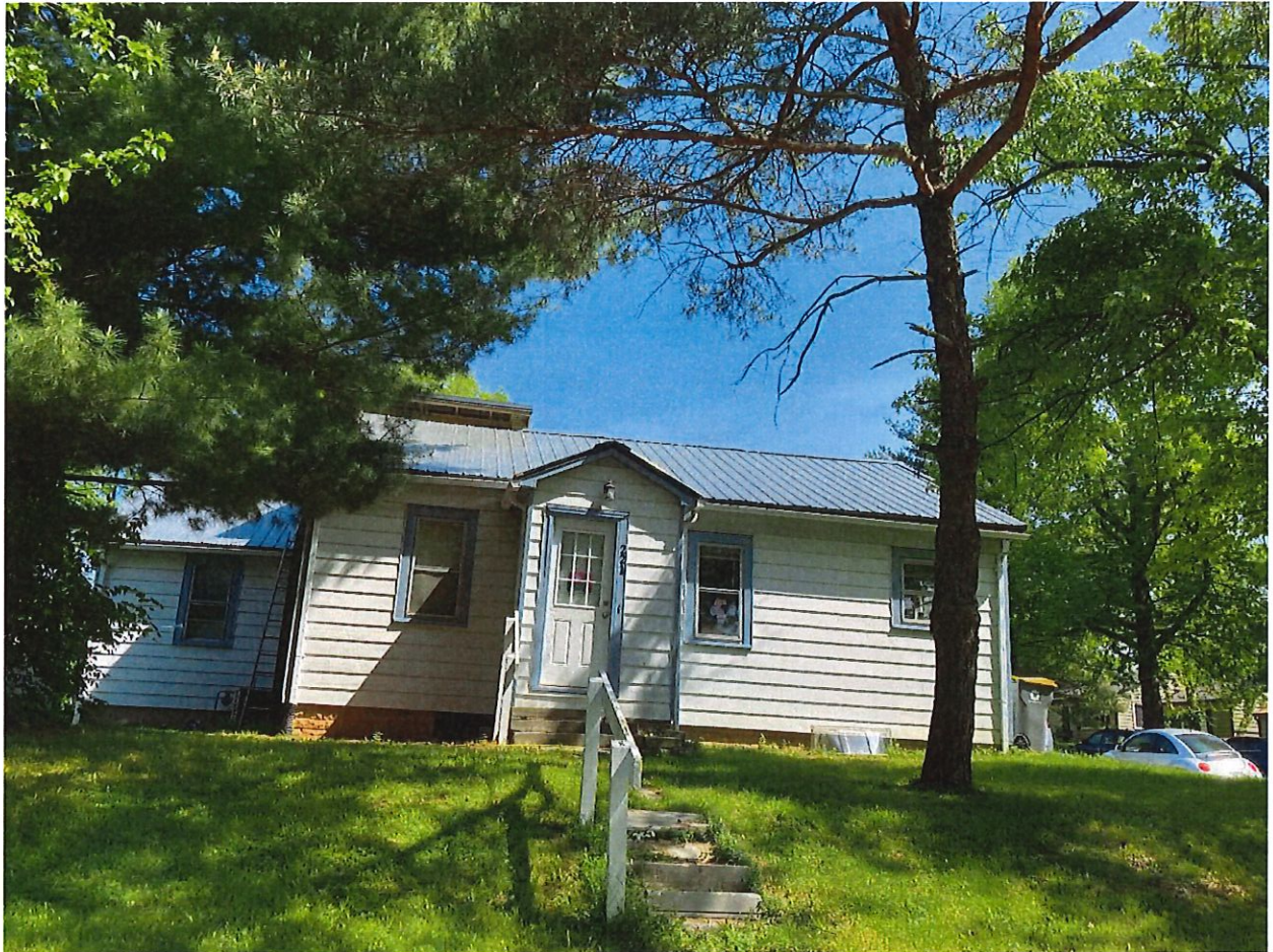
Photo 1: Roof of 221 E. Allen Street on 05/12/2022.
