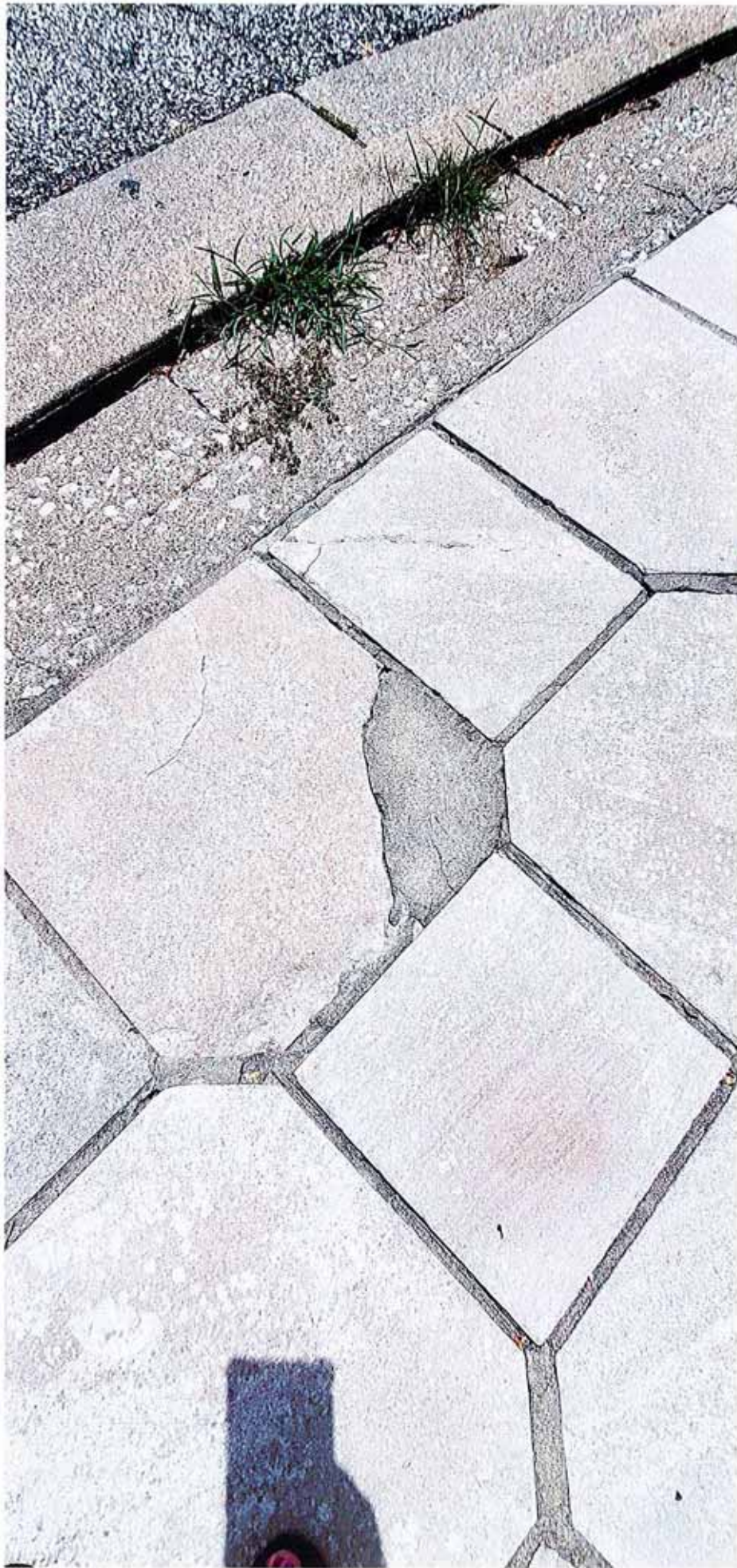
Rogers St WPA Sidewalk Repair
