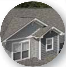
Roofing and Ventilation
