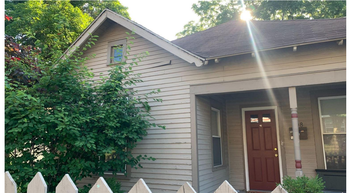
Image 12: West facade with the front entrance of the parsonage, bungalow, 2022 (photo by staff)
