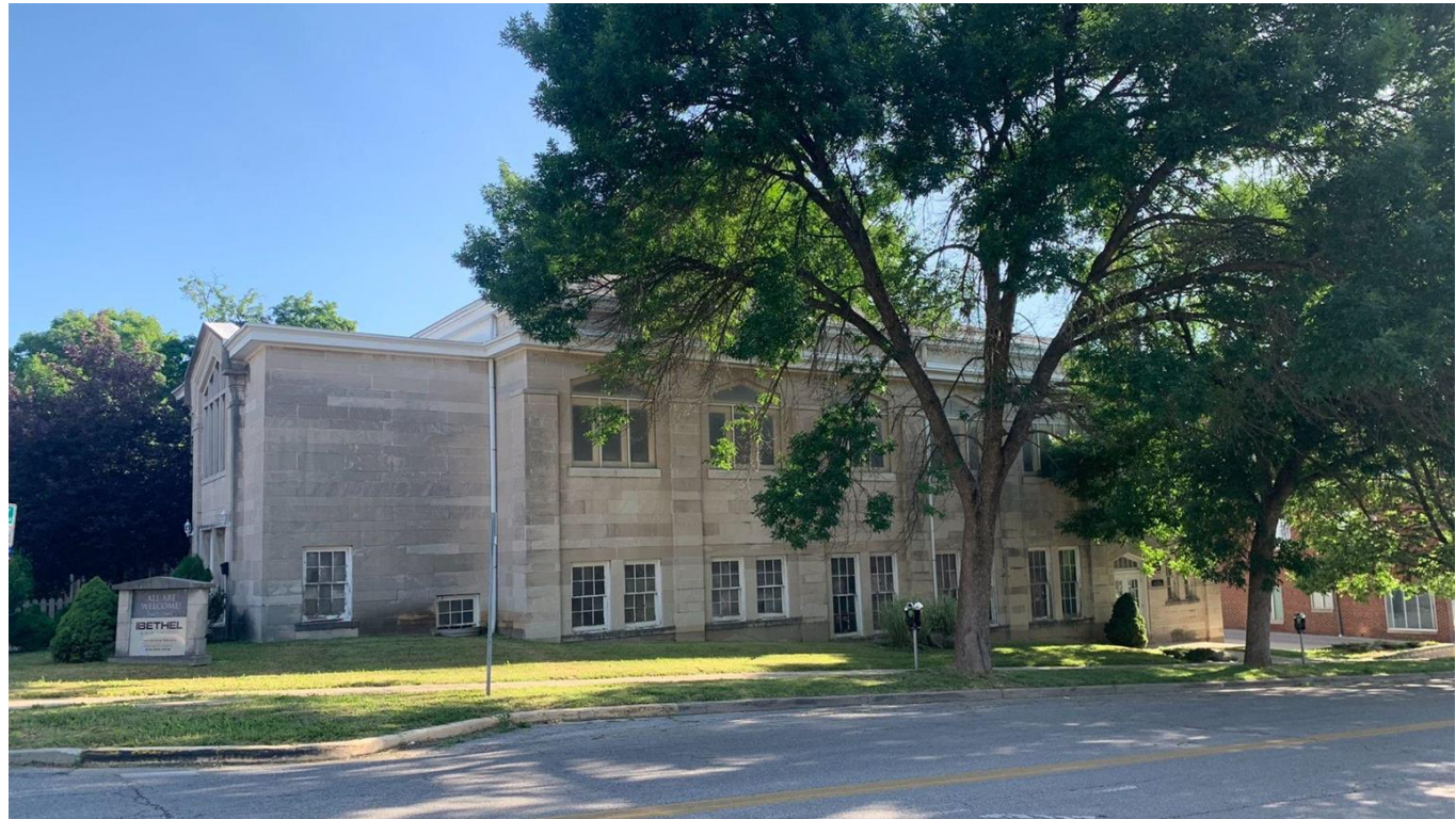
Image 7: Southern facade, showcasing six rows of windows, 2022 (photo by staff)
