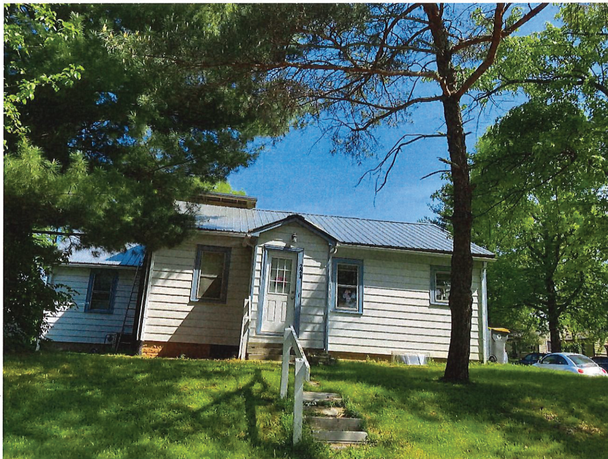
Photo 1: Roof of 221 E. Allen Street on 05/12/2022.
