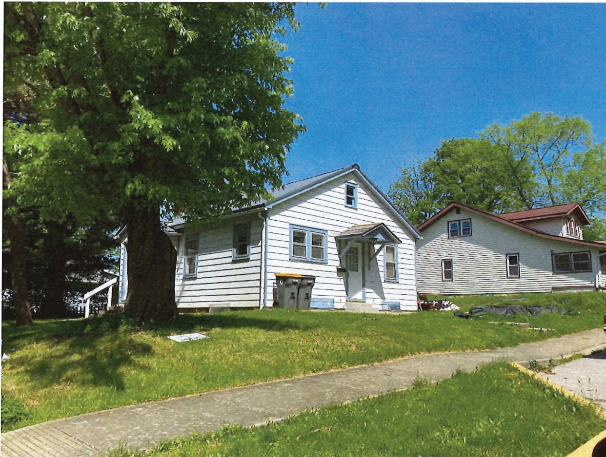
Photo 2: Roof of 221 E. Allen Street on 05/12/2022.
