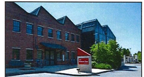
Plant #1 (west side)
