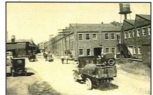
Plant #1 (looking south)
