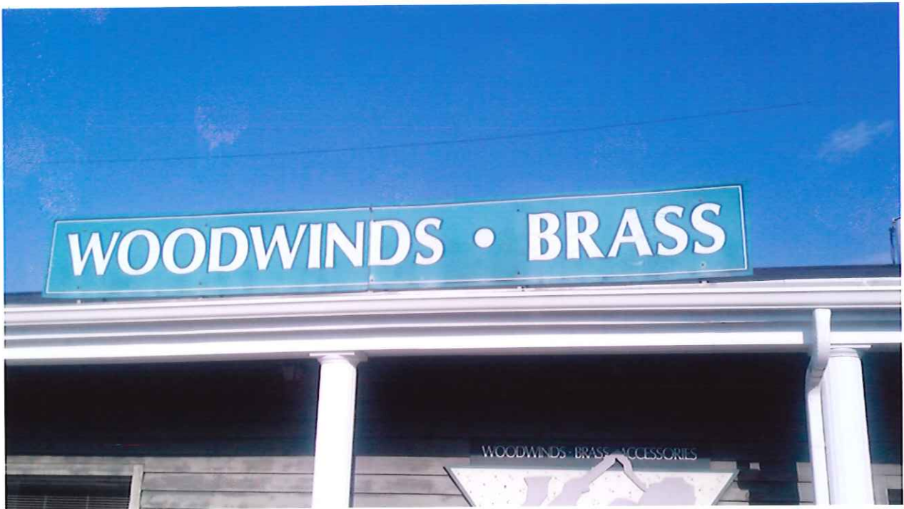
Remaining signage outdated, cracked, and faded
