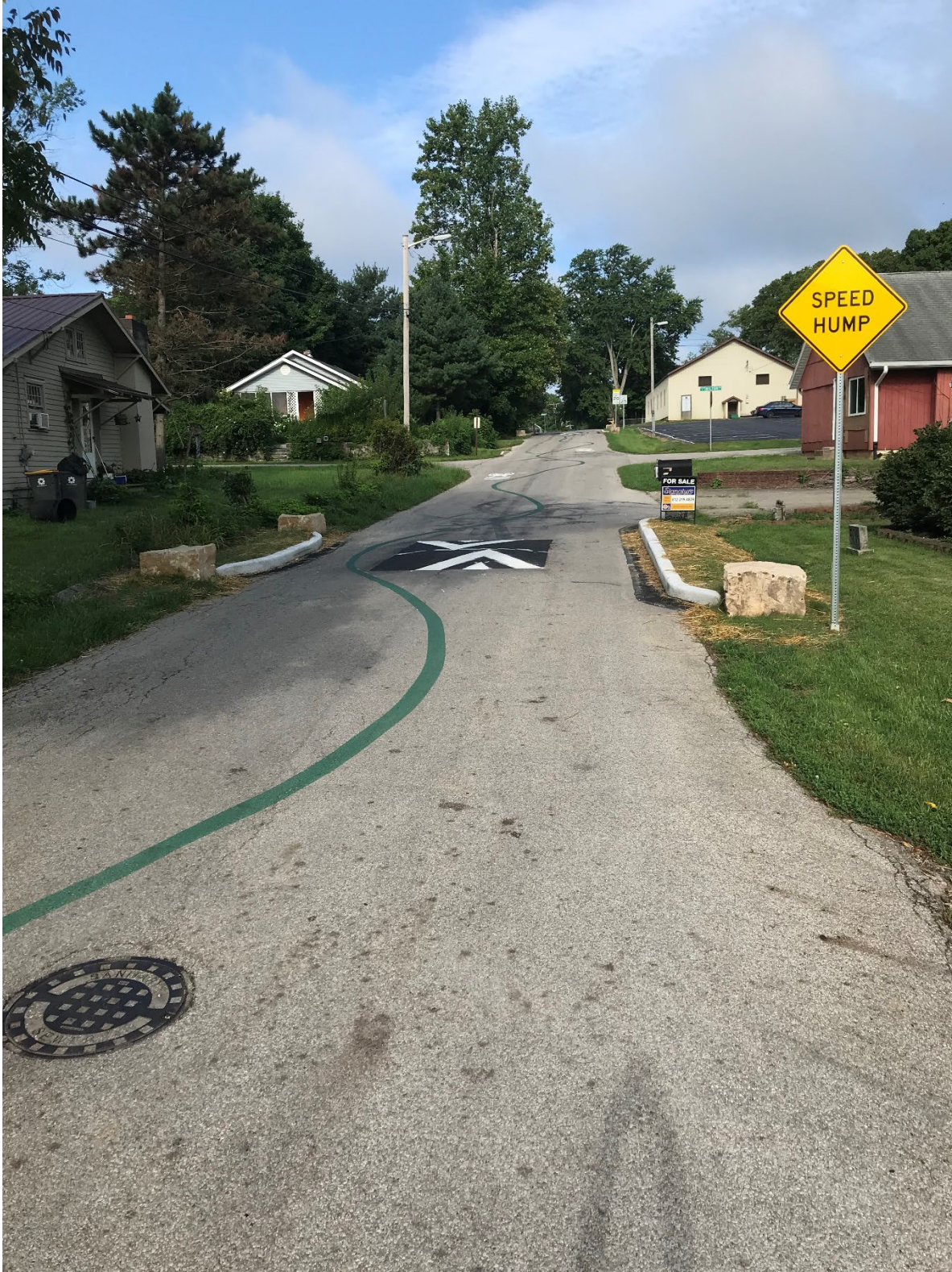
Image shows the Graham Street Neighborhood Greenway. There are shared lane markings, a speed cushion, concrete curbs that create a street edge, and a green painted line on the ground.
