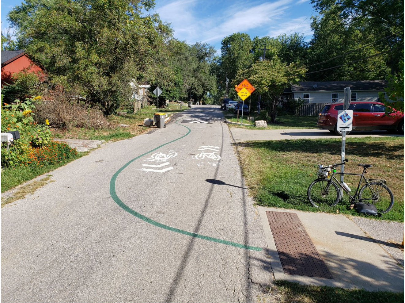
Image shows the Graham Street Neighborhood Greenway, where Bryan Street meets the trail that connects with the B-Line Trail. There are shared lane markings, a speed cushion, concrete curbs that create a street edge, and a green painted line on the ground.
