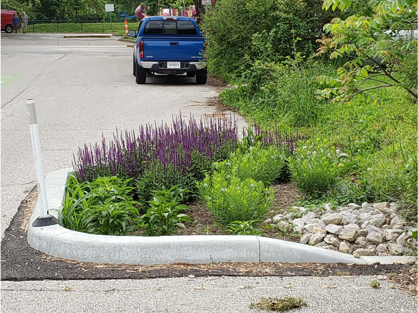
Image shows a bumpout into E. Allen Street with a concrete curb. The bumpout also serves as a raingarden, and includes plants that serve stormwater functions. This image is facing east, with Bryan Park visible in the background.
