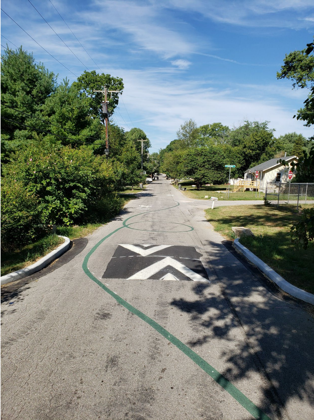
Image shows the Graham Street Neighborhood Greenway. There are shared lane markings, a speed cushion, concrete curbs that create a street edge, and a green painted line on the ground.
