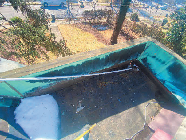
Copper to be removed and replaced with new 16 ounce copper
