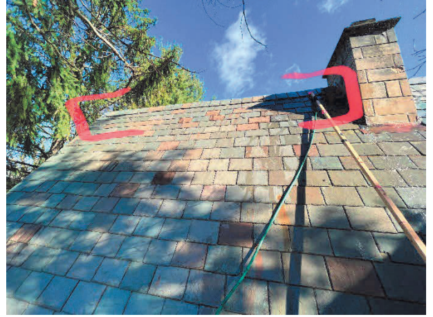
Ridge to be removed, flashing installed, slate re-installed – 16 ounce copper flashing
