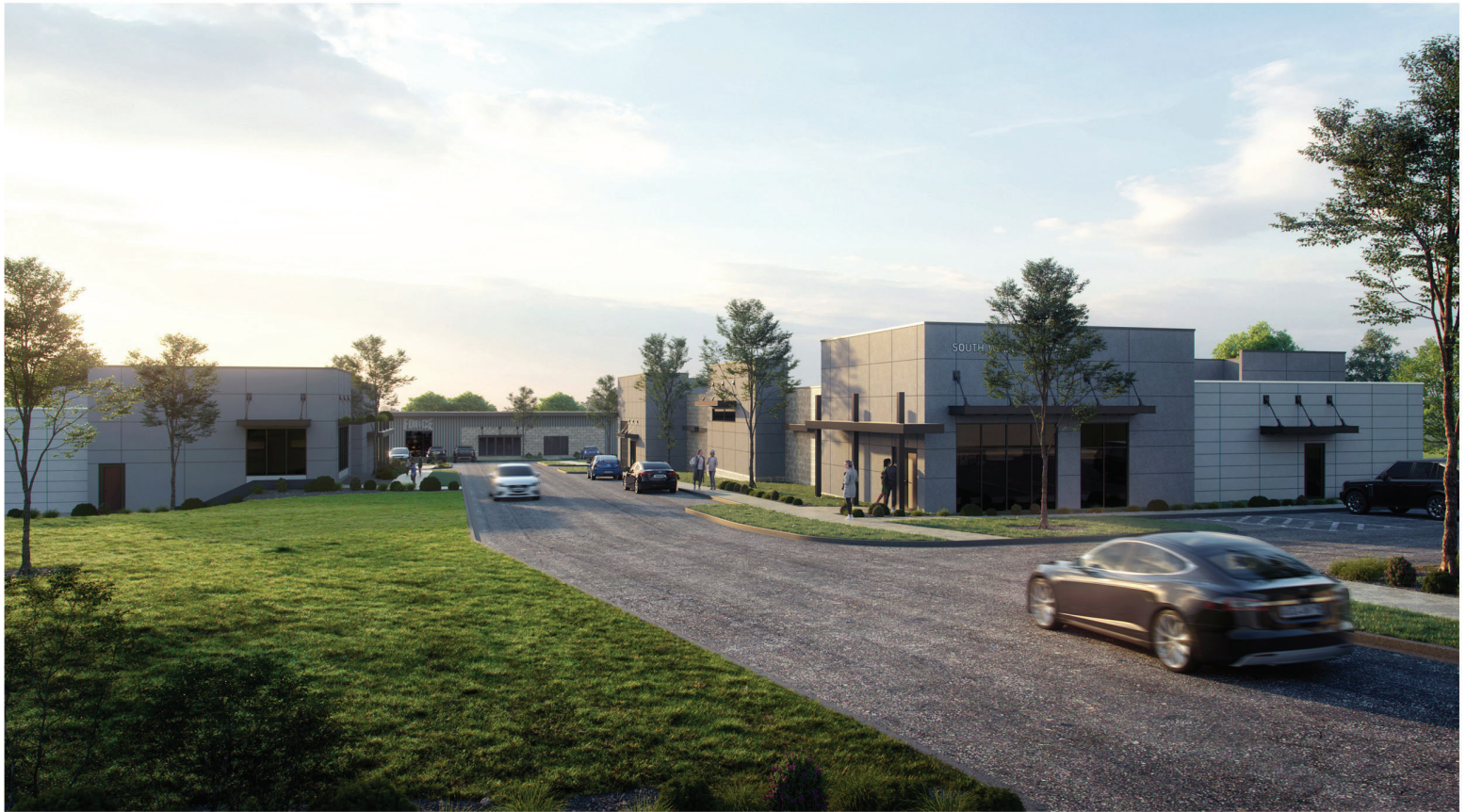
VIEW OF BUILDING #2 & BUILDING #3 LOOKING WEST
