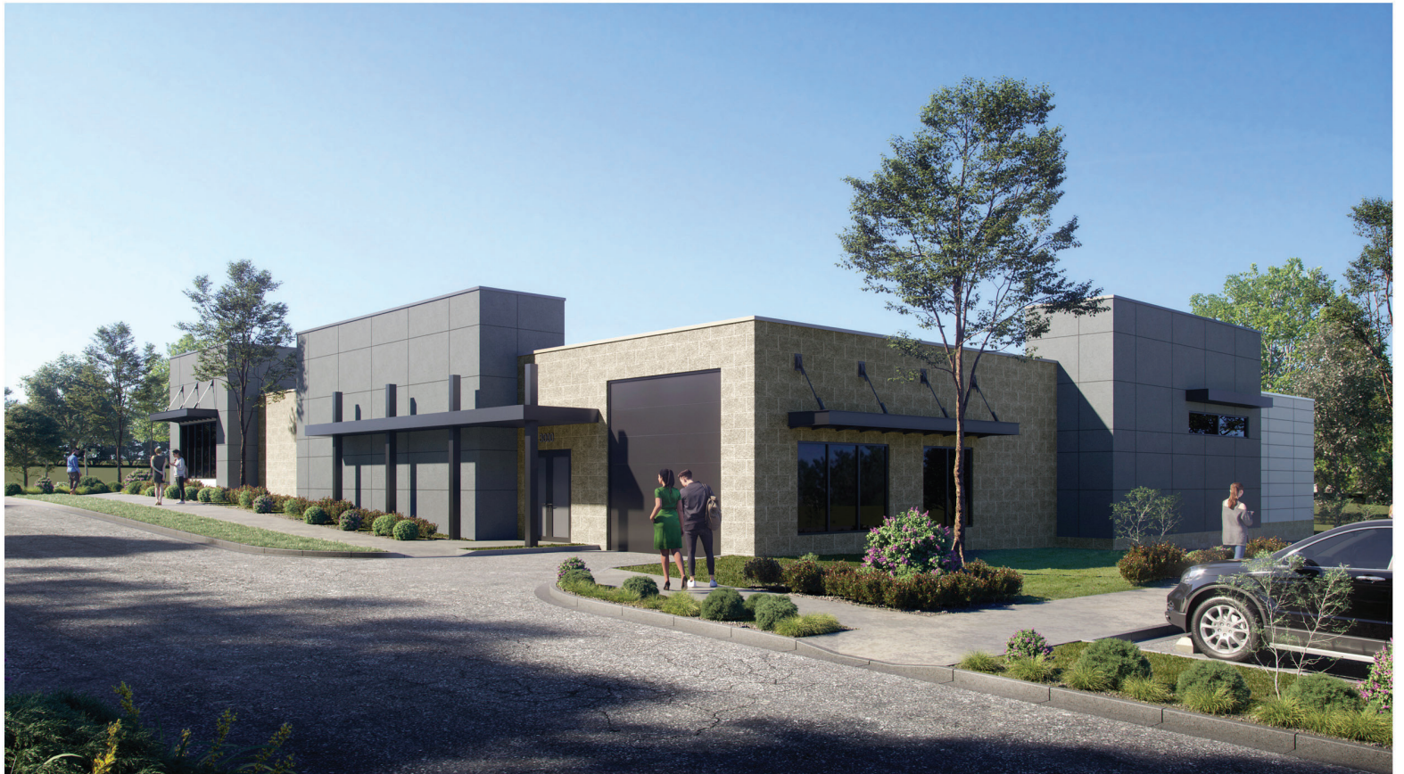
VIEW OF BUILDING #3 LOOKING SOUTHEAST
