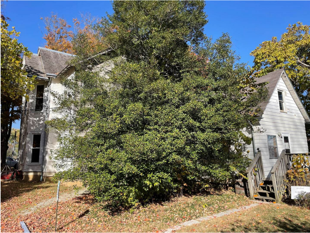
View of west and south sides of the house and woodshed addition
