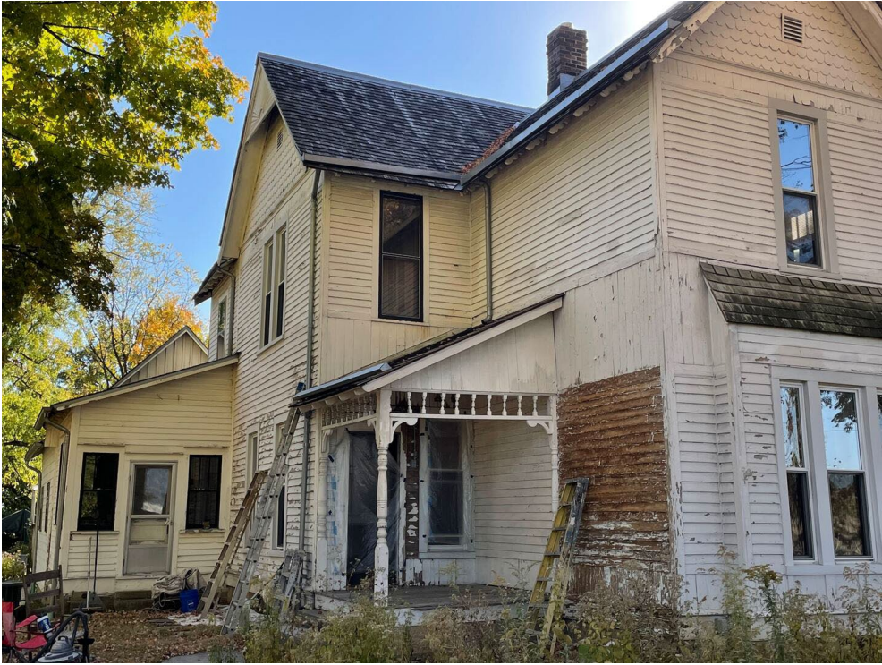
View of northeast side of the house
