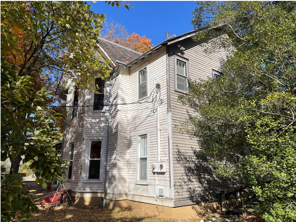
View of west and south sides of the house
