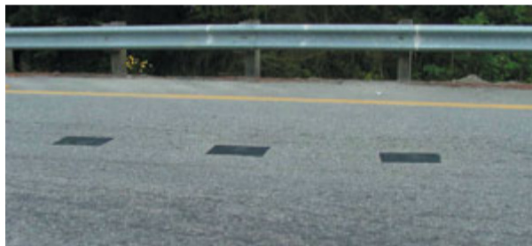
Electromagnetic sensors embedded in the pavement (the three dark squares) detect vehicles moving in the wrong direction (above).
