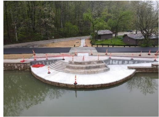
Griffy Lake Fishing Pier is now accessible.
