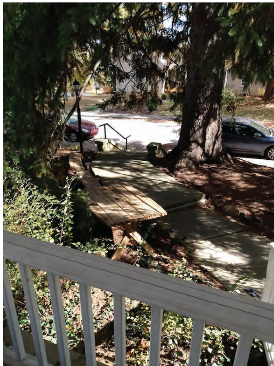
FIGURE 5. Alternate view of walkway in need of railing (on the left side of walkway in the photo).
