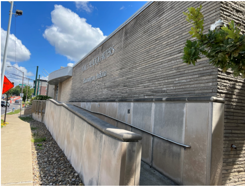
FRONT ENTRY (PUBLIC) RAMP
