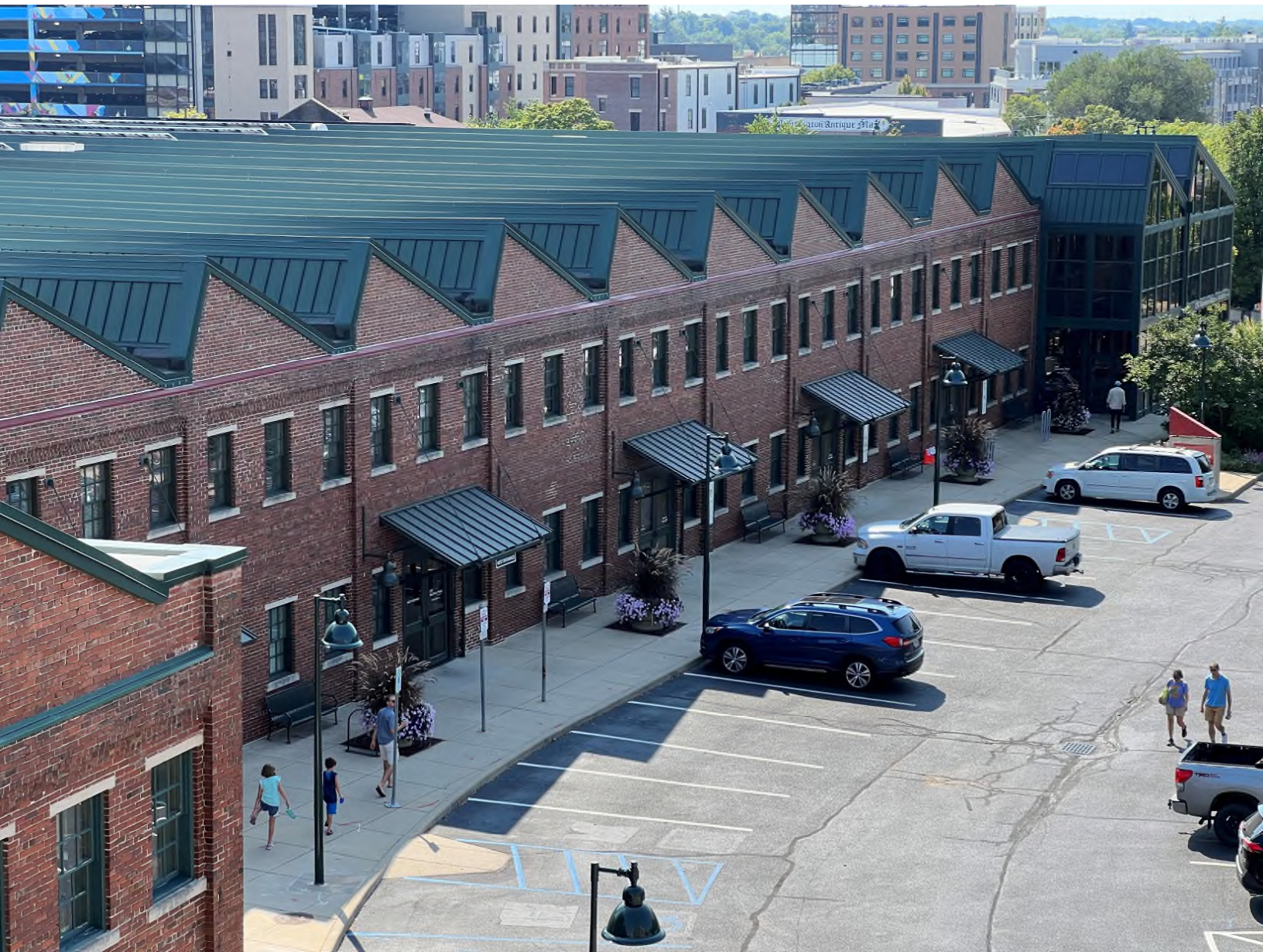
CFC Showers Building
