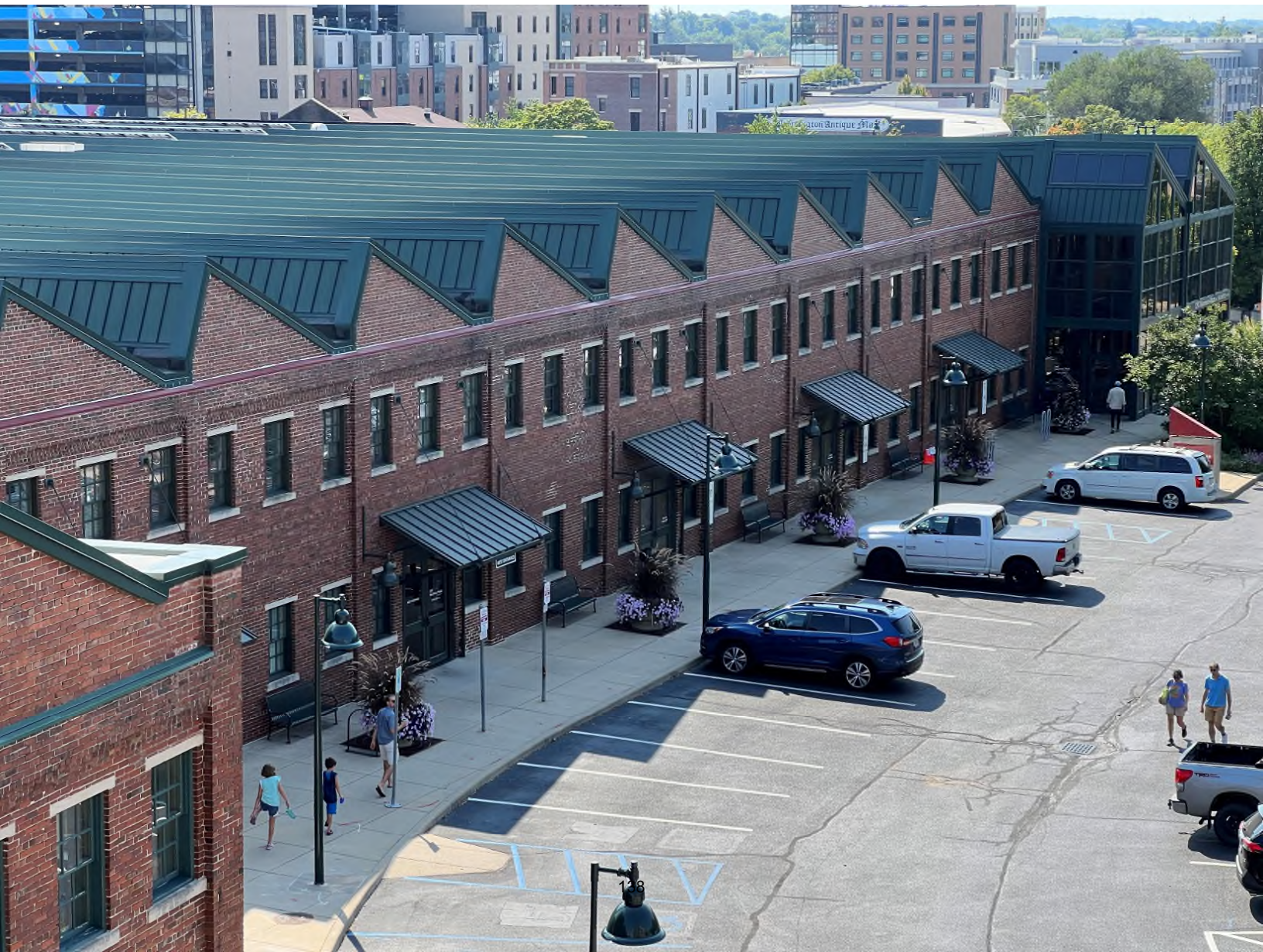
CFC Showers Building
