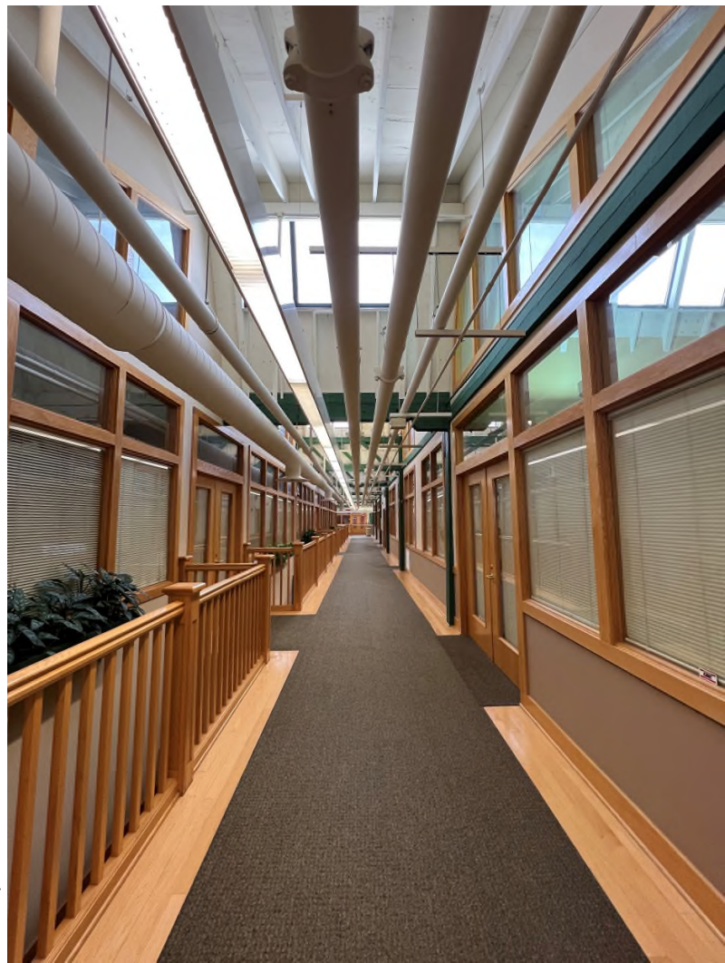
Interior Circulation with Roof Monitors
