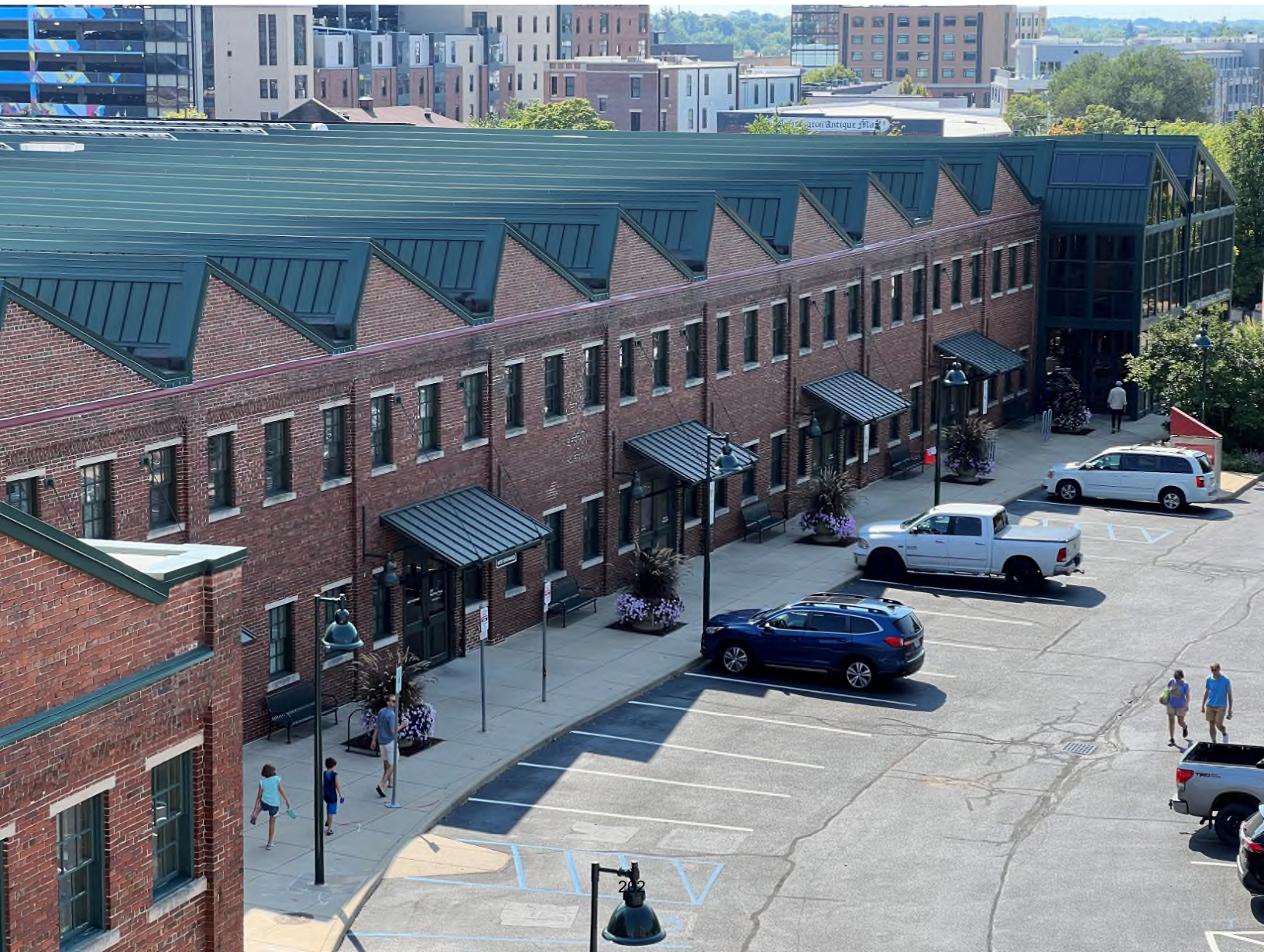
CFC Showers Building
