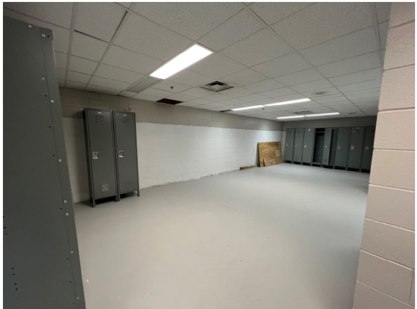
LOCKER ROOM (POST FLOOD)
