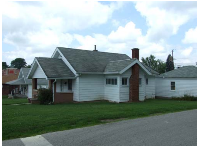
Typical California bungalow E 14 th Street
