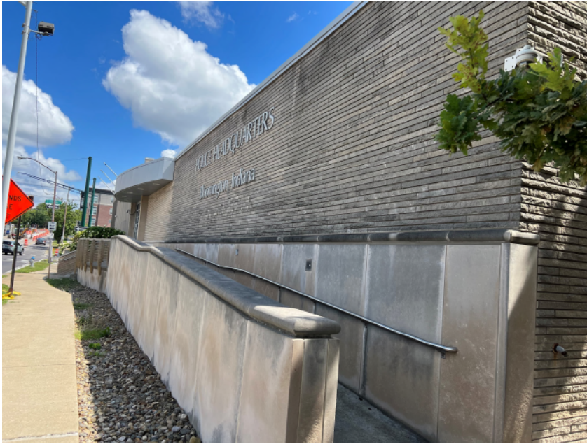
FRONT ENTRY (PUBLIC) RAMP
