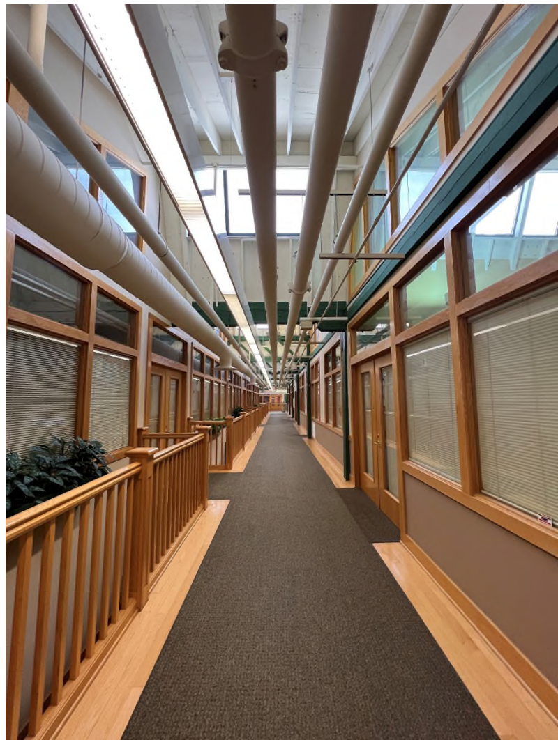
Interior Circulation with Roof Monitors
