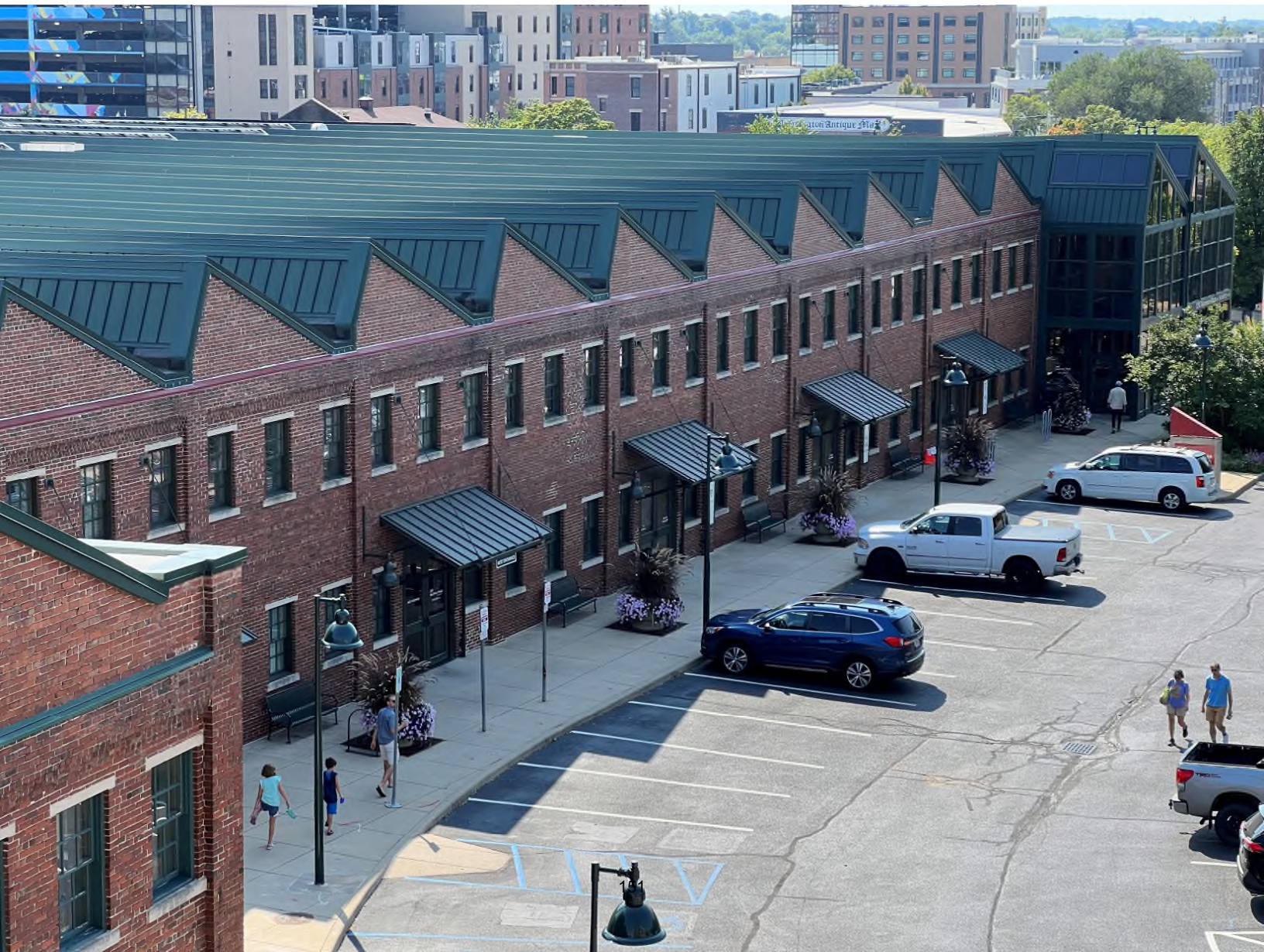
CFC Showers Building
