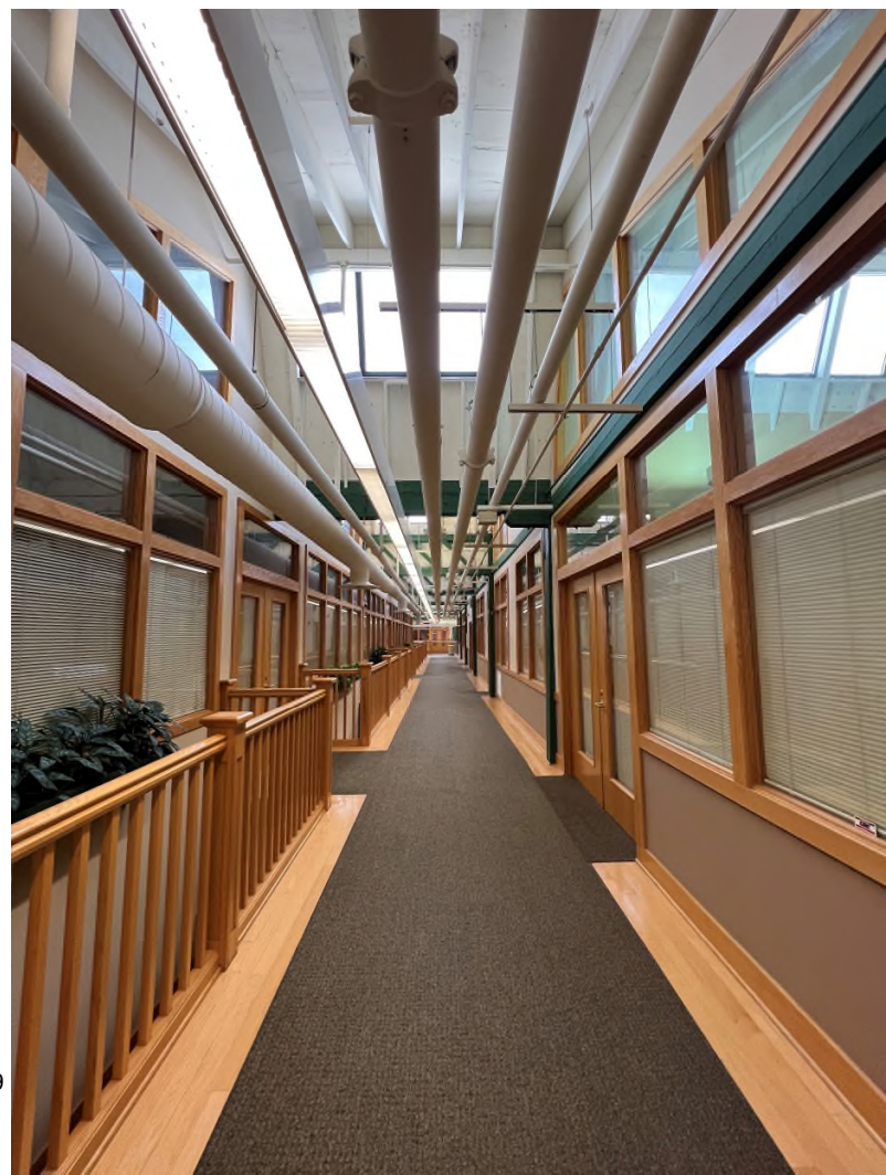
Interior Circulation with Roof Monitors
