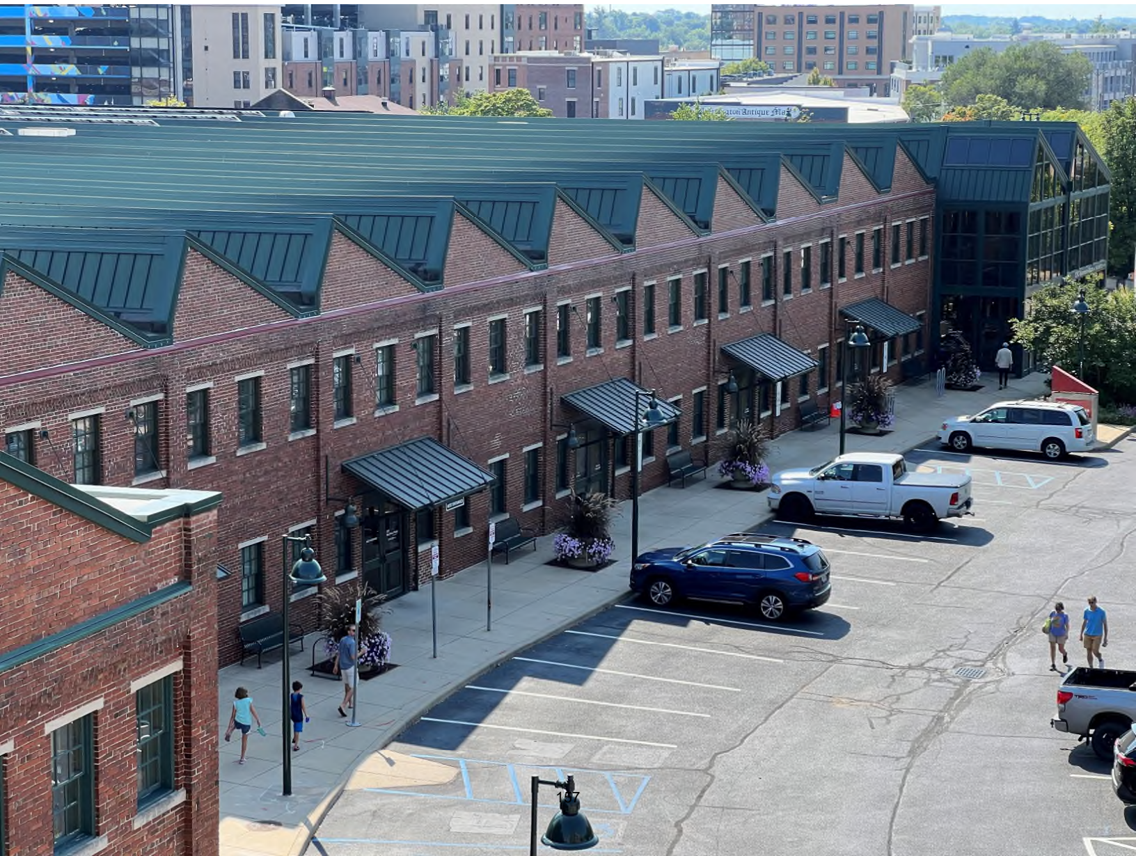
CFC Showers Building
