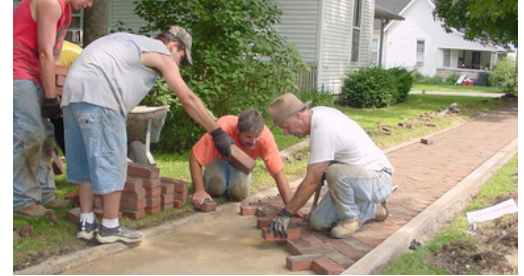
Bryan Park historic brick sidewalks restoration
