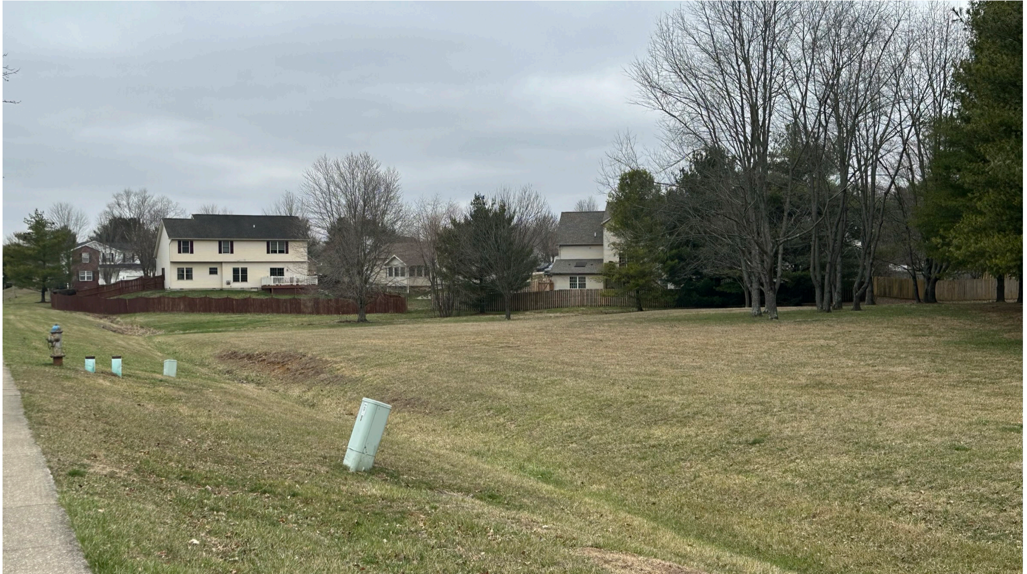
Bioretention Pond Site 1 - Facing south.
