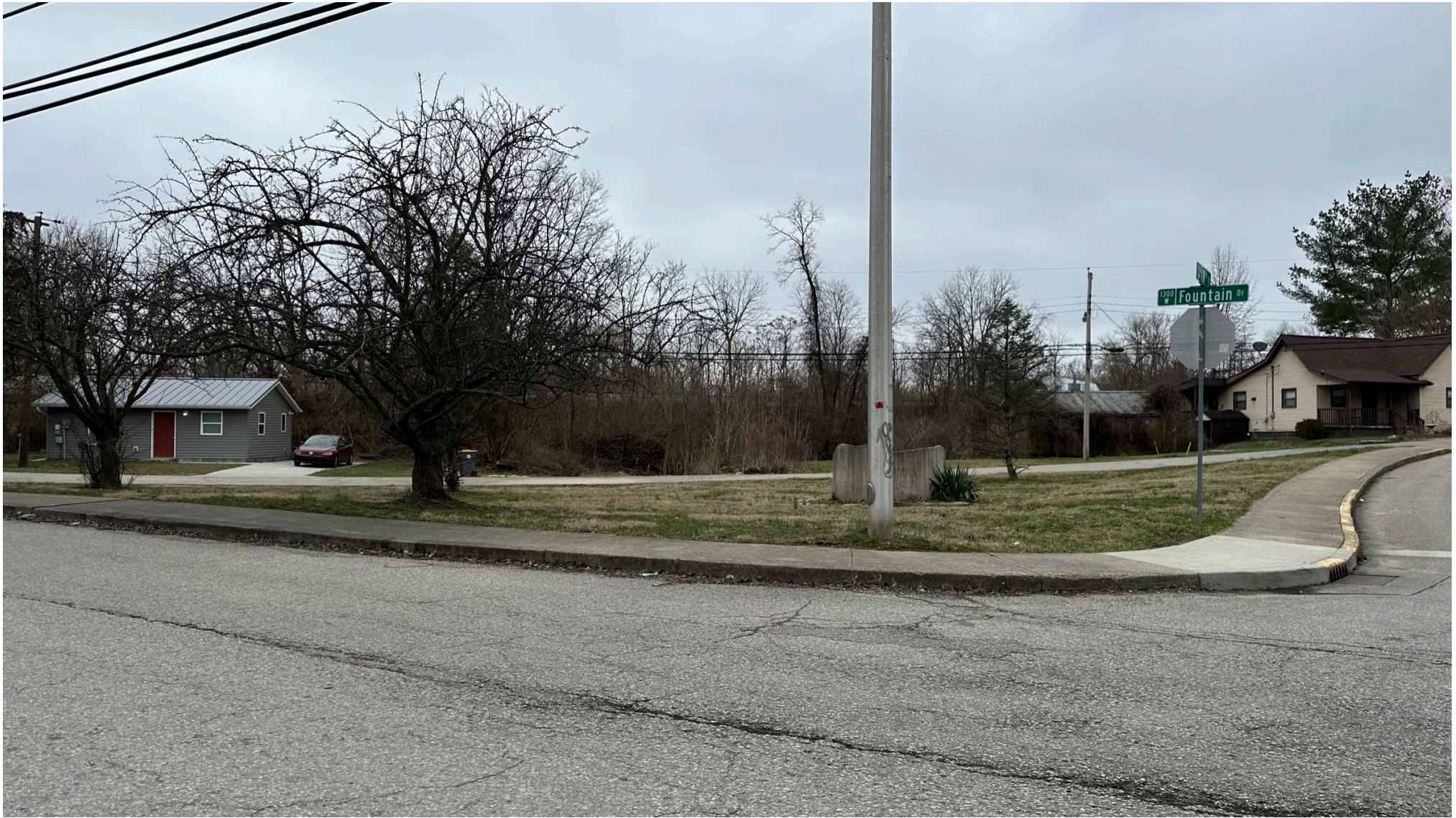
Bioretention Pond Site 3 - facing northwest
