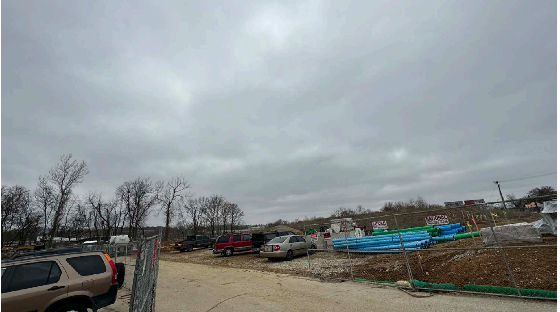
Retreat at Switchyard Facing northwest into the project site (March 1, 2023)
