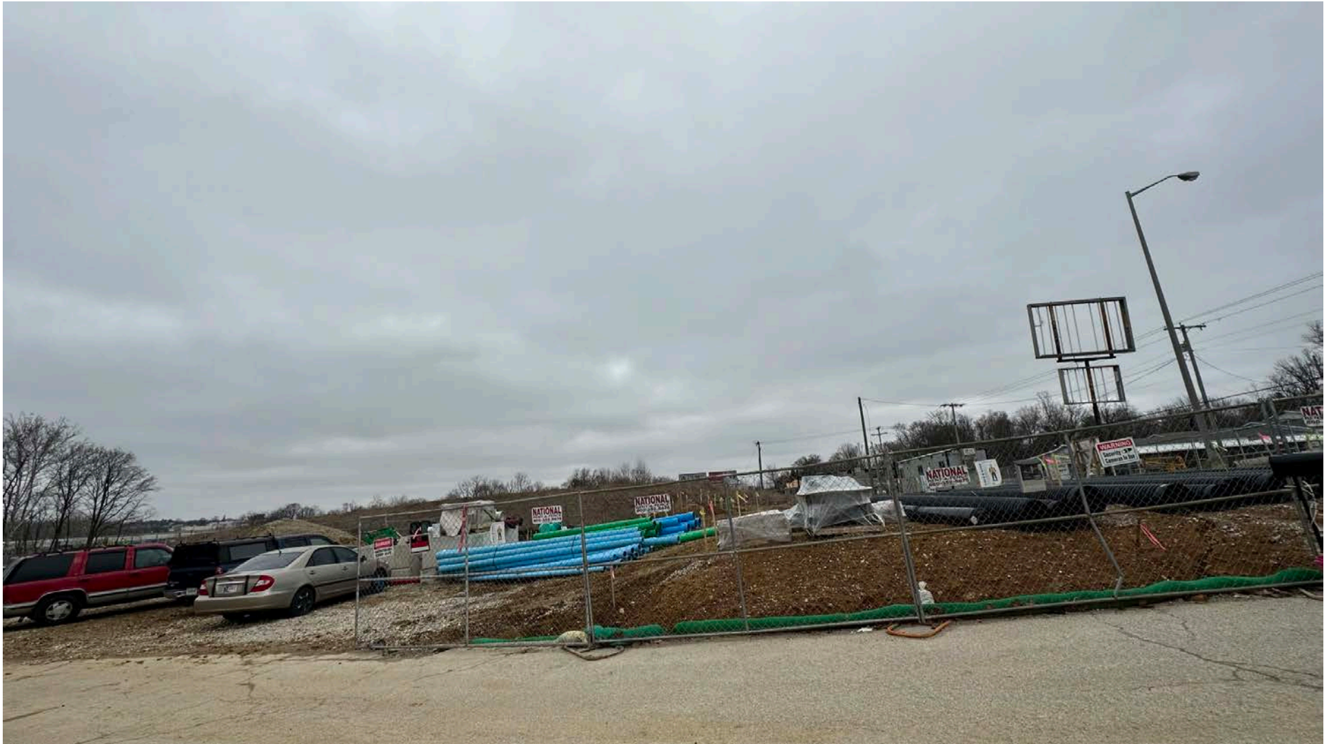
Retreat at Switchyard Facing northward into the project site (March 1, 2023)
