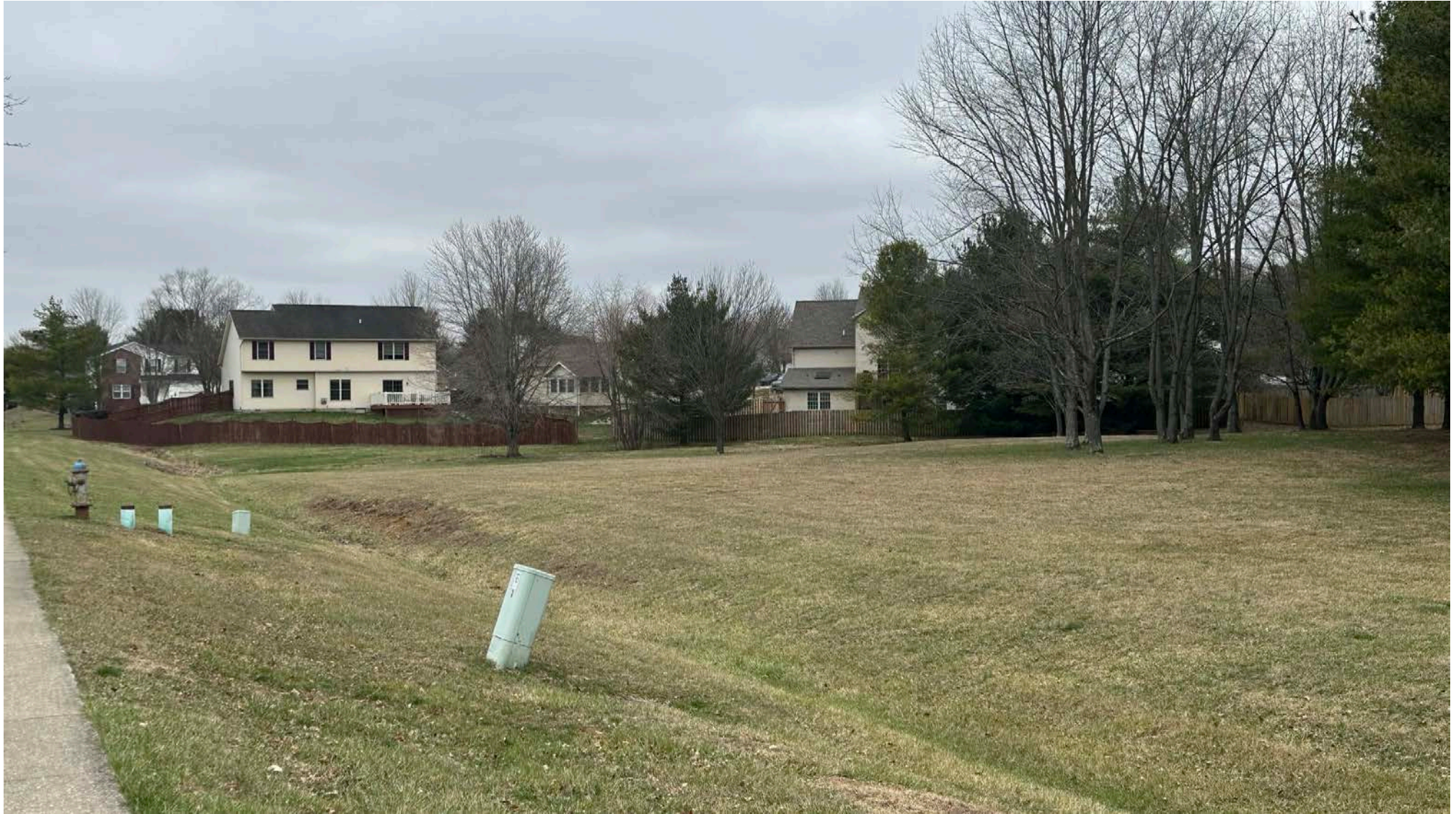
Bioretention Pond Site 1 - Facing south.
