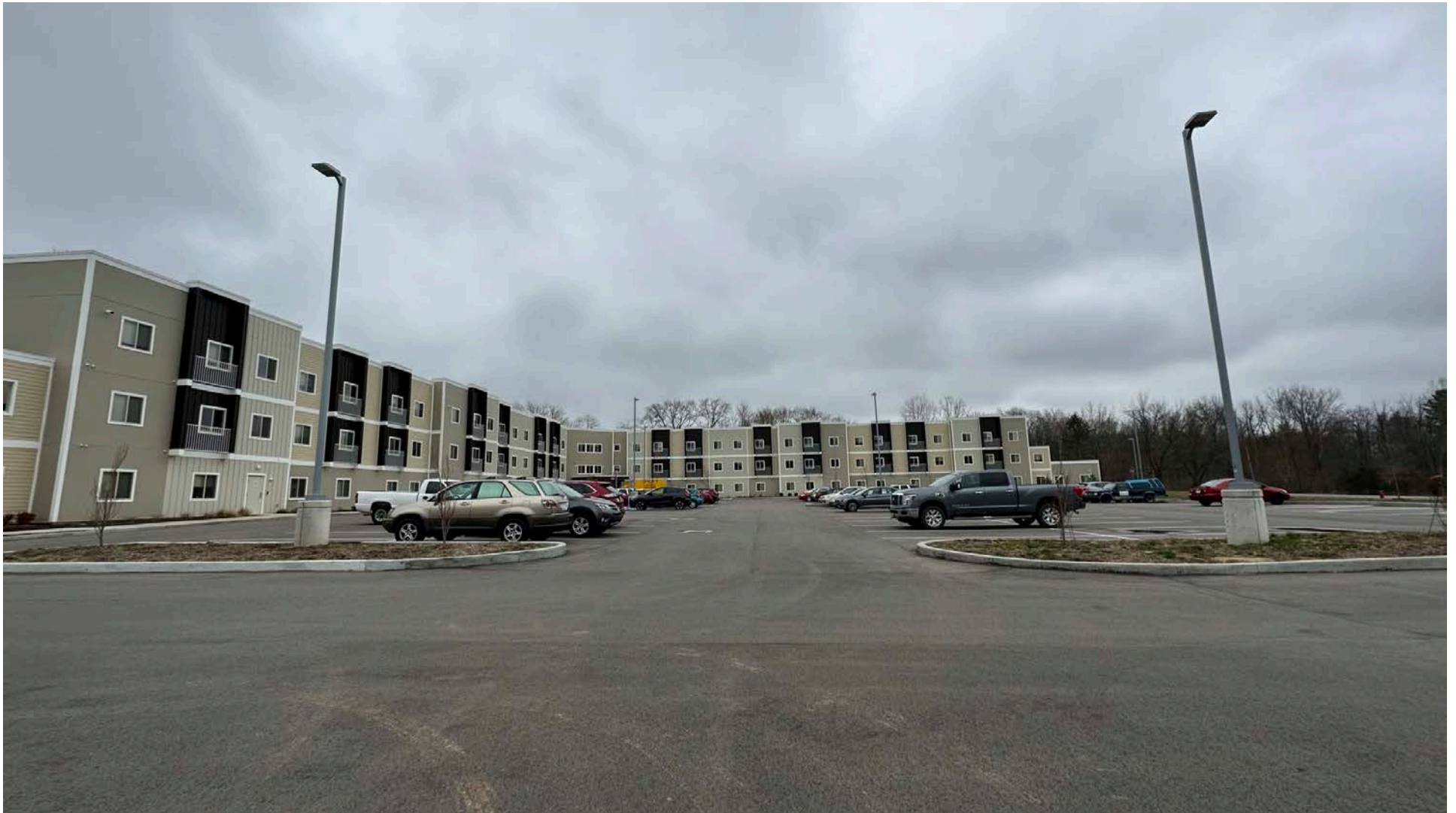
Photo 1 - facing northeast towards the main building (2023).
