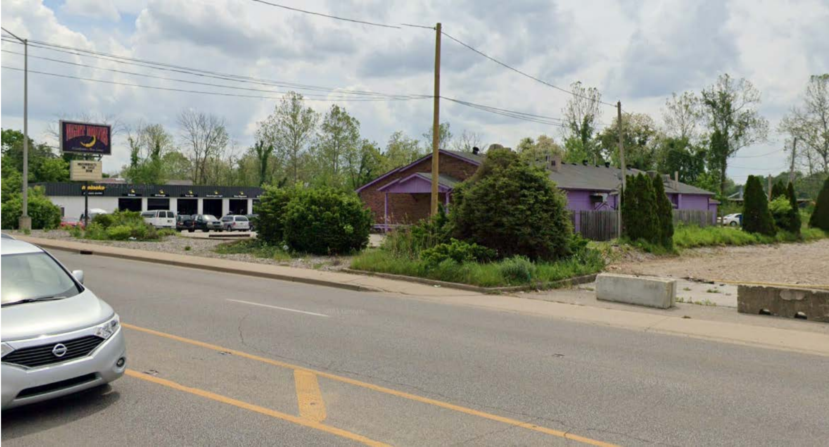
Image of building on site that has been demolished. (Image from Google Maps)
