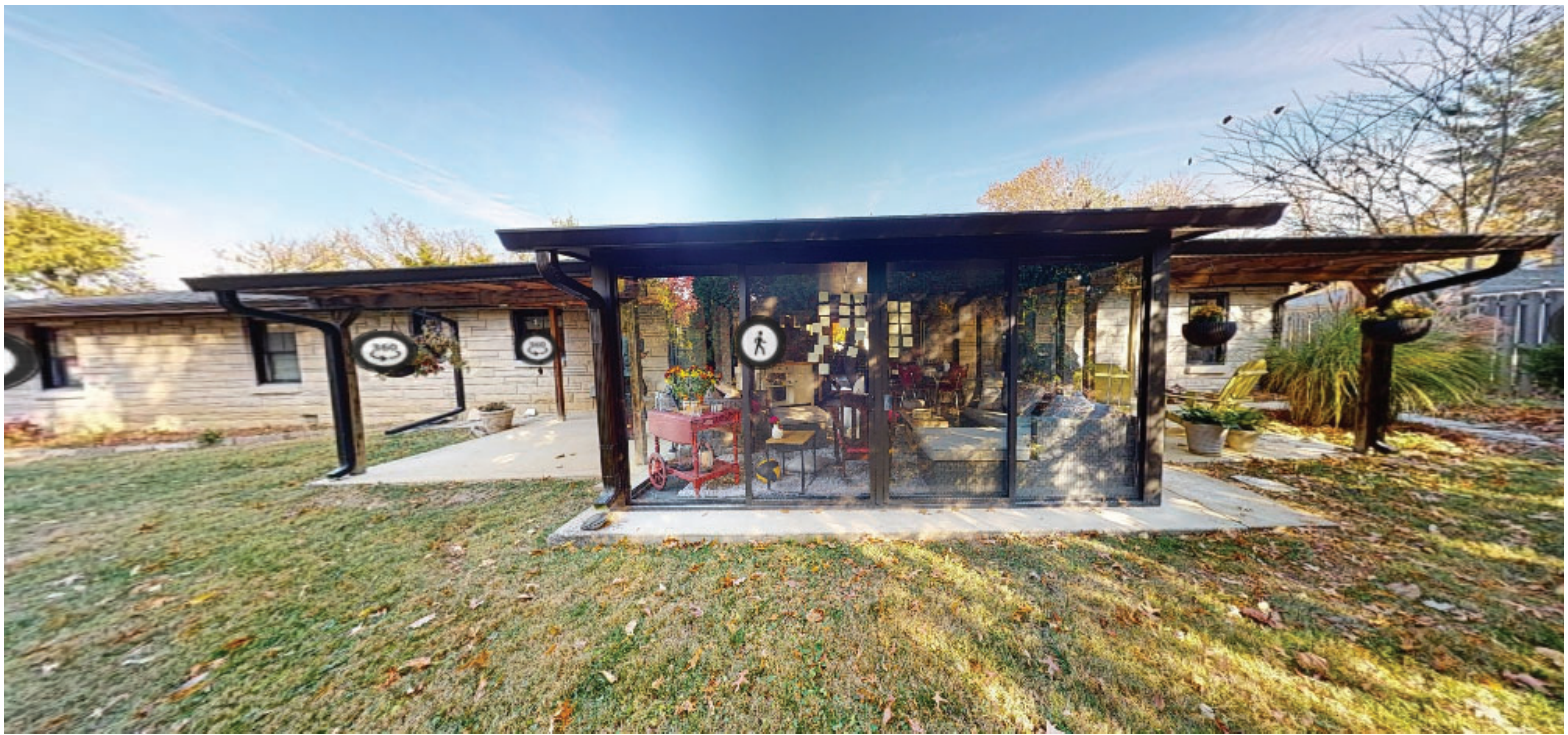
LOOKING NORTH, EXISTING THREE SEASONS ROOM
