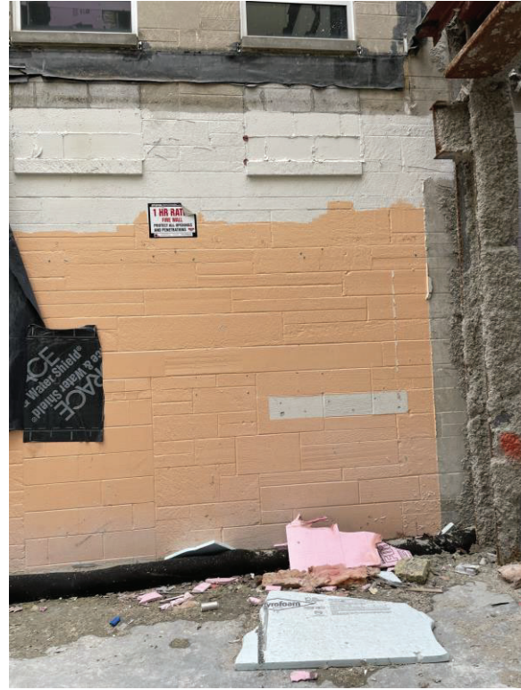
Photo 13. Lower Section of North Elevation
