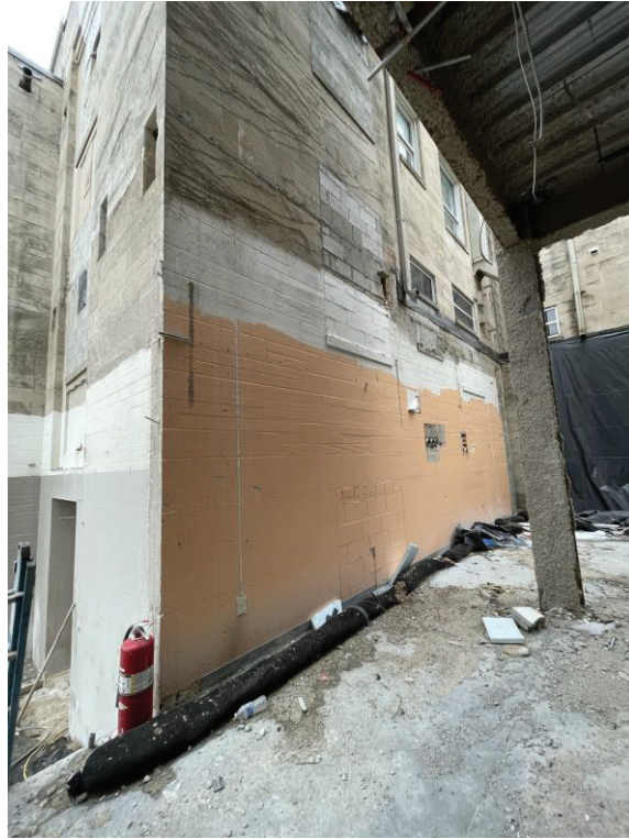
Photo 9. Lower Area of West Elevation
