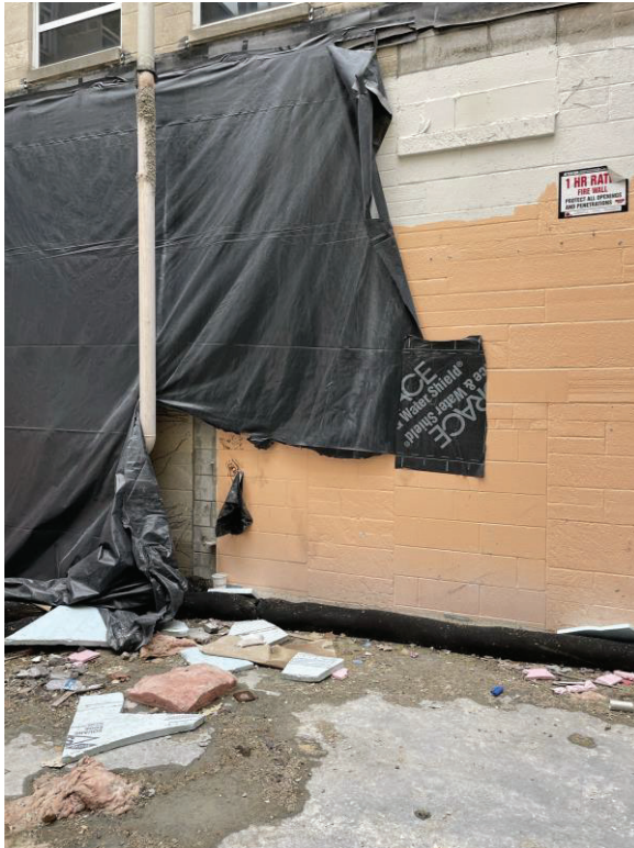
Photo 14. Lower Section of North Elevation
