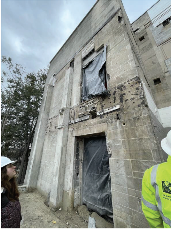
Photo 4. North Stair, Integrated Concrete Columns
