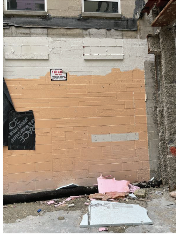
Photo 13. Lower Section of North Elevation
