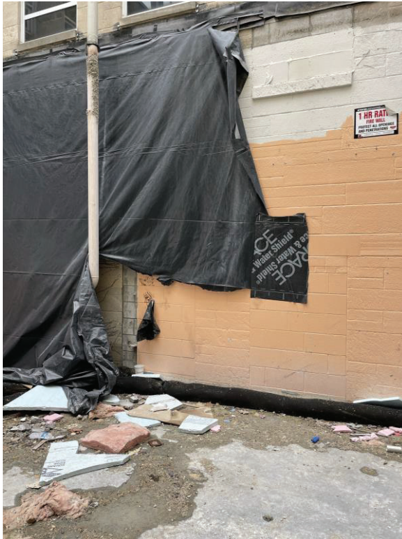
Photo 14. Lower Section of North Elevation
