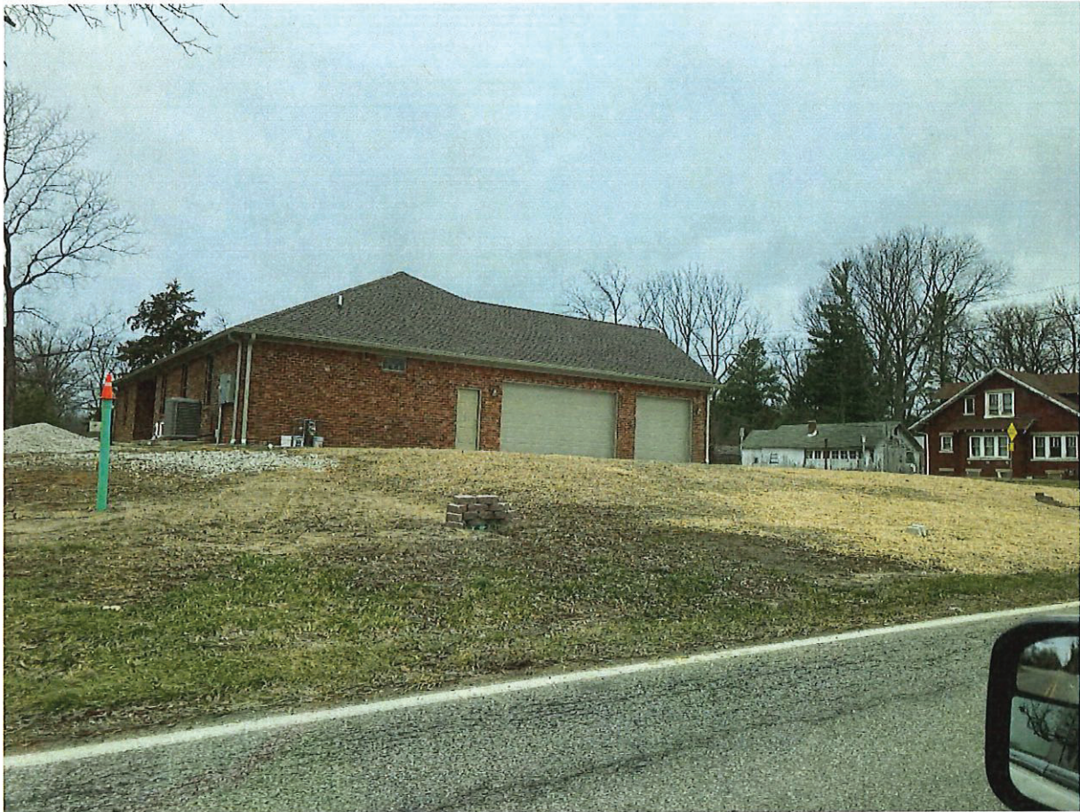
Photo 1: The portion of the 2028 E 1 st Street site adjacent to High Street where a sidewalk and tree plot have not yet been built on 02/14/2023.
