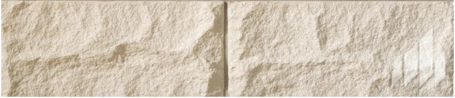
BELOW WINDOW SILL
