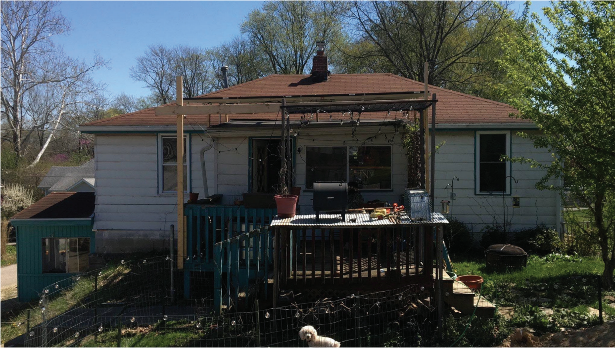
looking EAST at existing main structure
