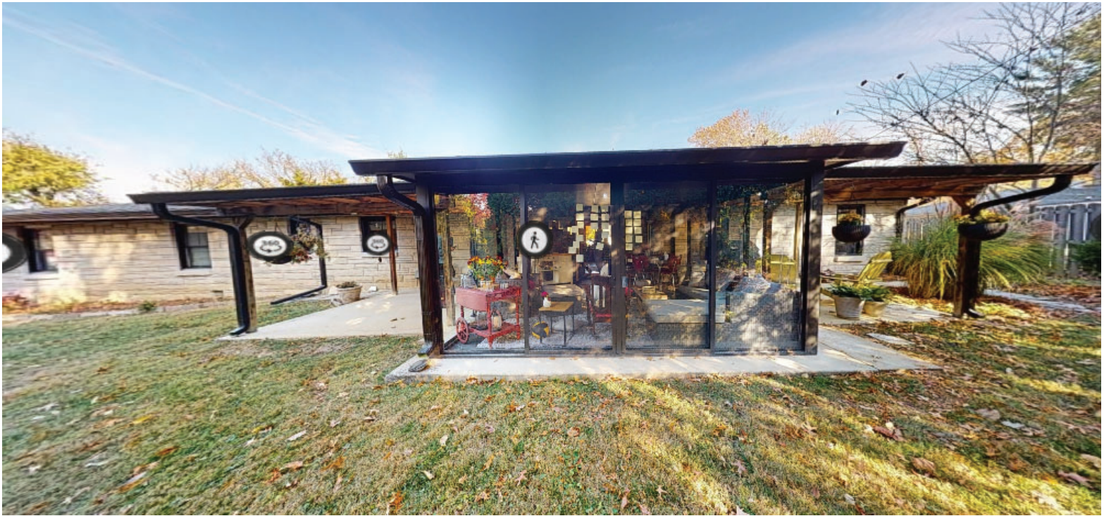
LOOKING NORTH, EXISTING THREE SEASONS ROOM
