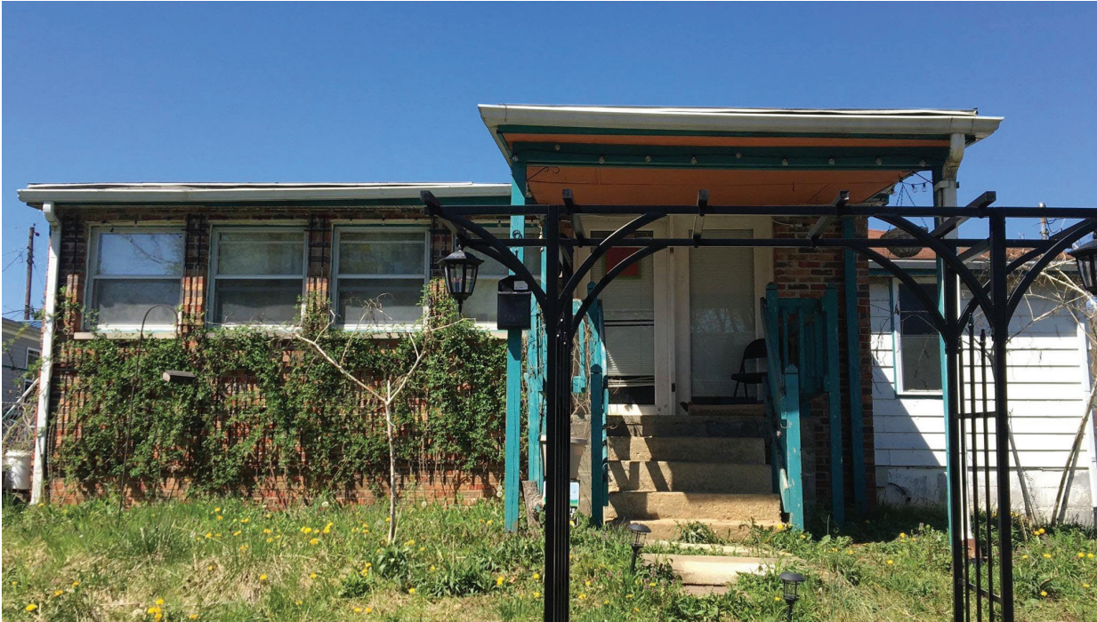
façade from Fairview looking EAST
