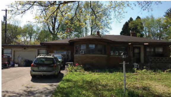
1105 N Woodburn Ave view II
