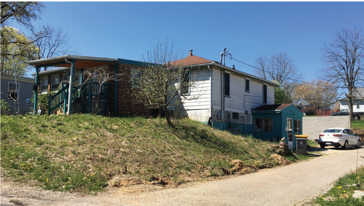
façade from Fairview and alley intersection, looking SOUTHWEST
