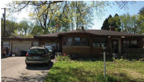
1105 N Woodburn Ave view II
