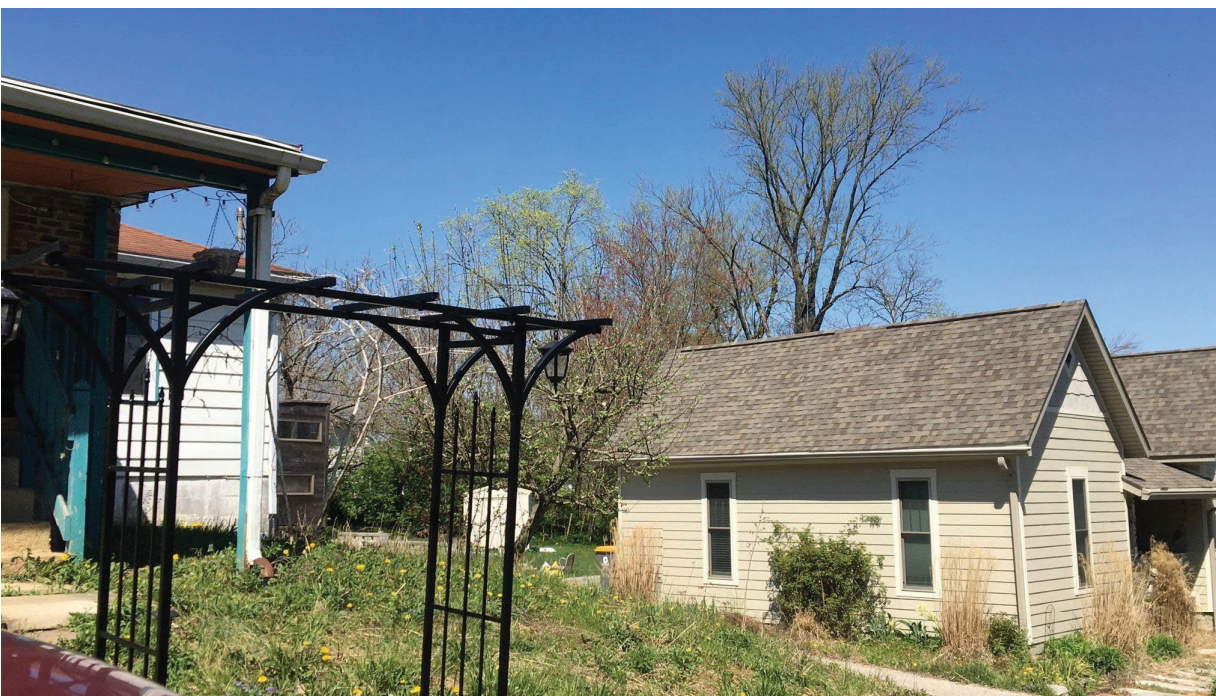
façade from Fairview, showing northern neighbor, looking NORTHWEST
