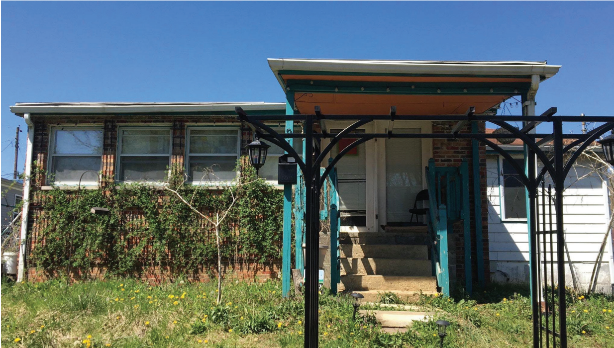
façade from Fairview looking EAST
