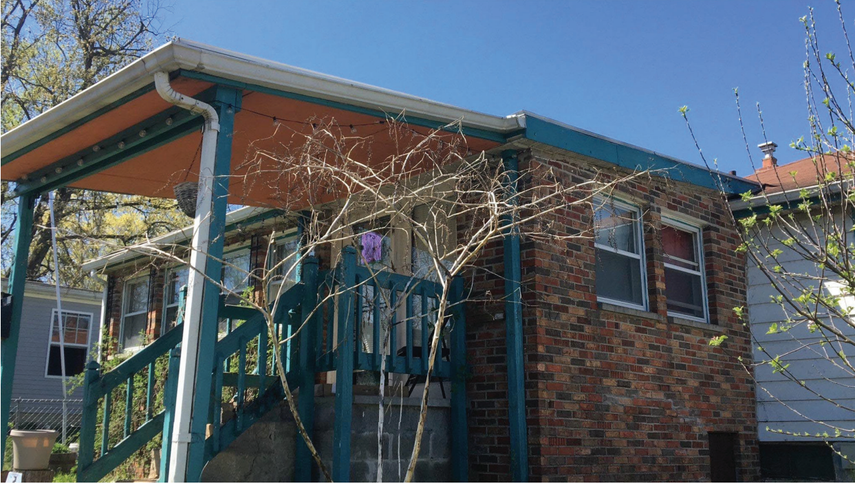
façade from Fairview, looking SOUTHWEST
