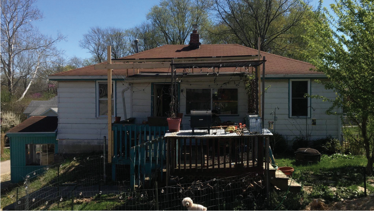
looking EAST at existing main structure
