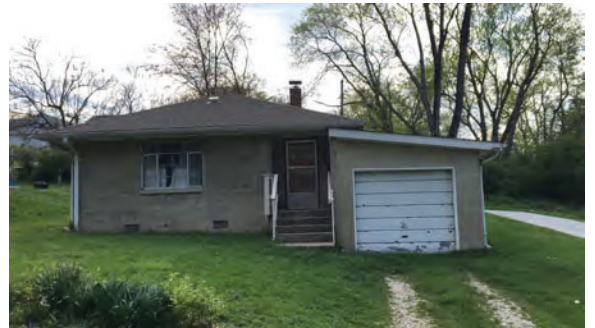
931 N Fairview St
