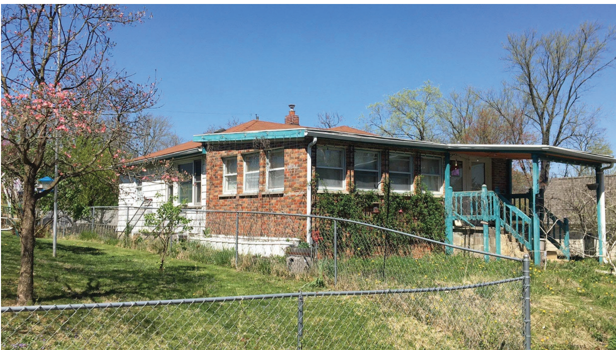
façade from Fairview, looking NORTHWEST
