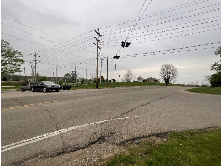
Southeast corner looking Northwest at overhead electric lines crossing Old SR 37
