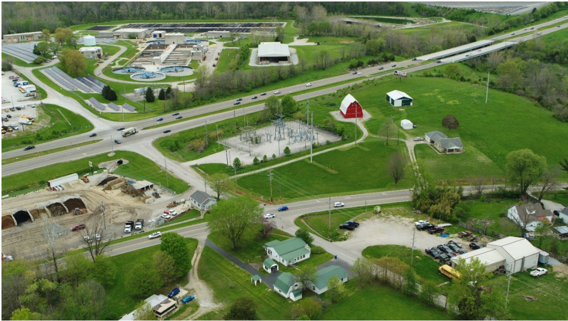
Overhead Aerial View of Old SR 37 at Dillman Road looking Northwest
