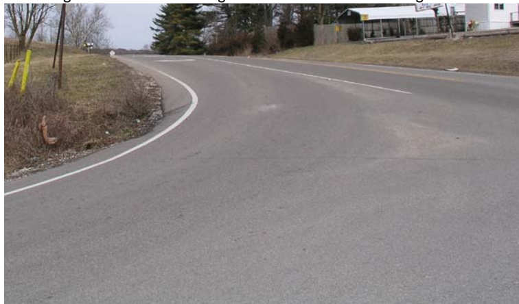
Figure 1: On west leg of intersection looking north
