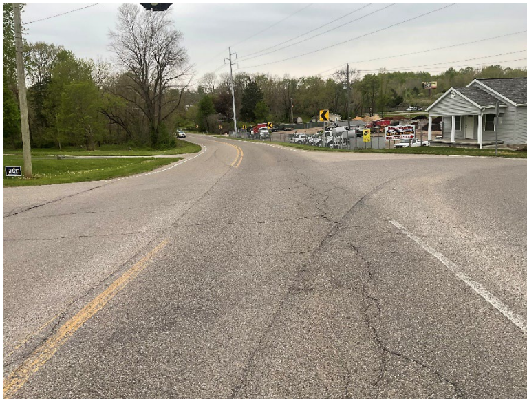
Old SR 37 at Dillman Road intersection looking South
