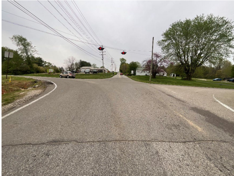
Old SR 37 looking North at the intersection with Dillman Road
