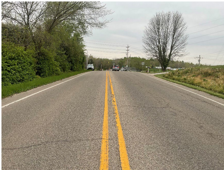
Old SR 37 looking South towards intersection showing sight distance problem
