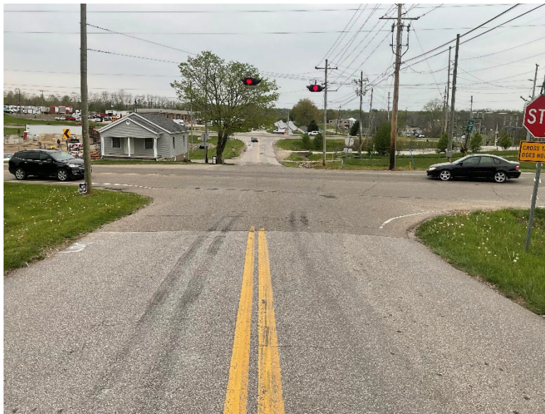
Dillman Road Eastbound approach to Old SR 37 showing grade change along Dillman Road
