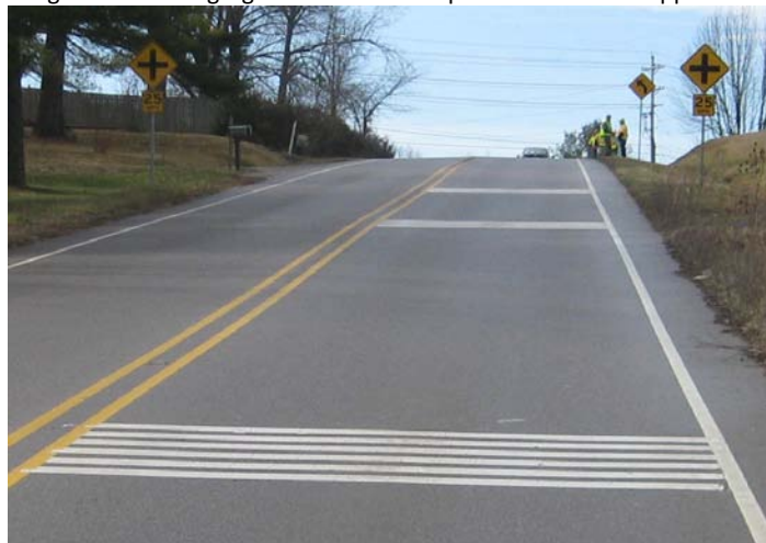
Figure 3: Warning signs and rumble strips on southbound approach
