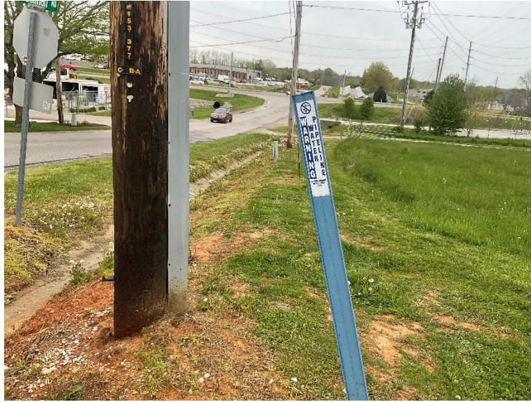
Water Pipeline Marker Northwest Quadrant of intersection
