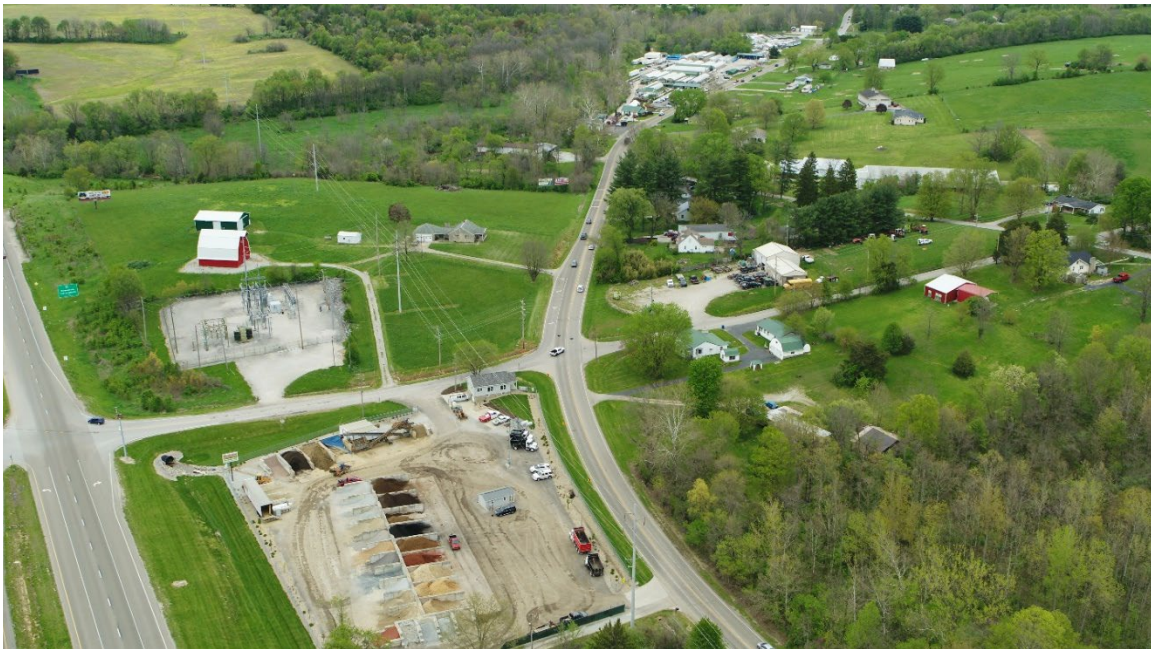
Overhead Aerial View of Old SR 37 at Dillman Road looking Northeast
