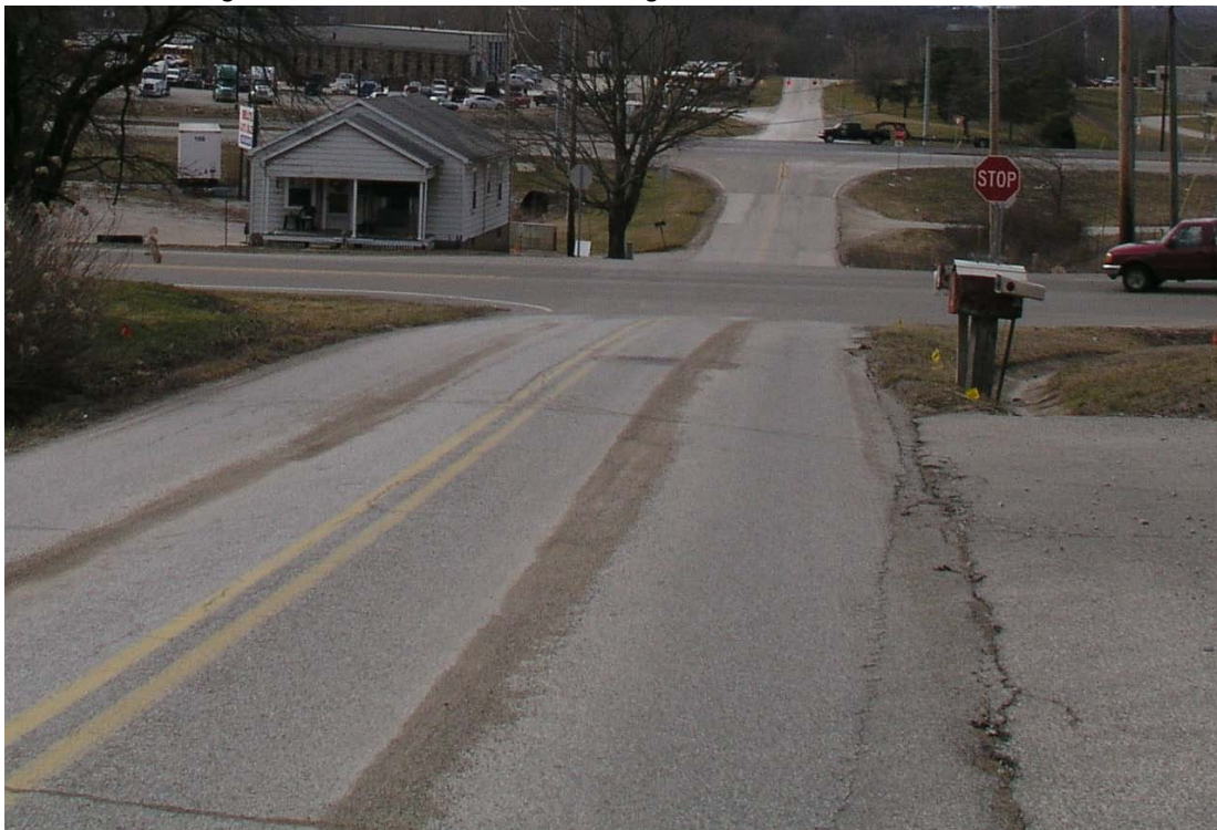
Figure 9: On Dillman Road looking west towards intersection
