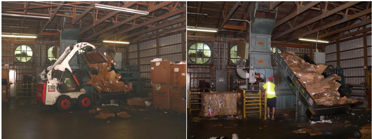
Monroe Co. SWMD's old baler purchased by Martin Co. SWMD over fifteen years ago still up and running. Albertson indicated that they have virtually no mechanical problems with their balers.
