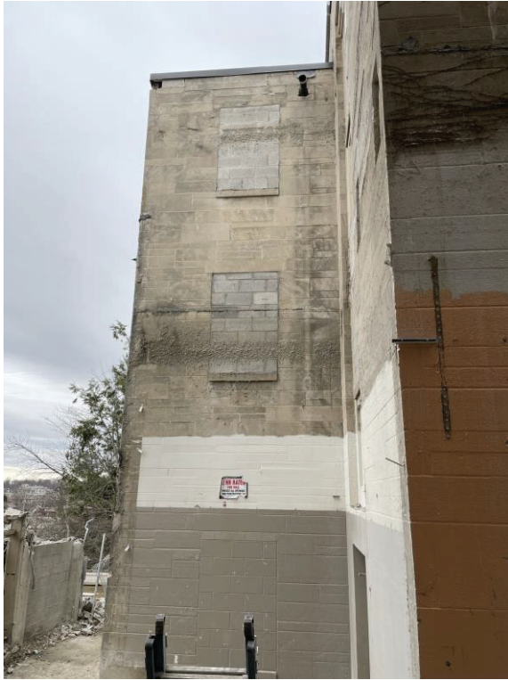
Photo 8. West Elevation of North Stair
