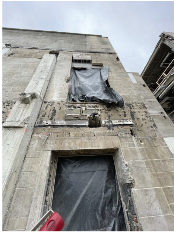
Photo 5. North Stair, Former Door & Glass Block Opening
