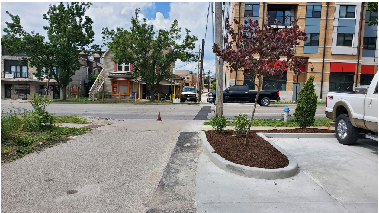
Looking north to E. Third St. from the alley
