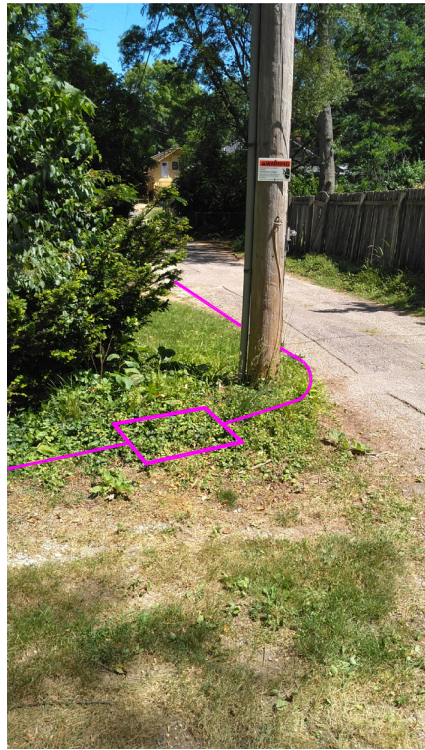
PROPOSED LINEAL UH2X3 GROUND ROD/BUS BAR LEAVE 50' TAIL BFO24 SEQ. IN _____ SEQ. END _____ TELECOM LEAVE 50' TAIL SEBO12 FLAT SEQ. END _____ SEQ. OUT _____
