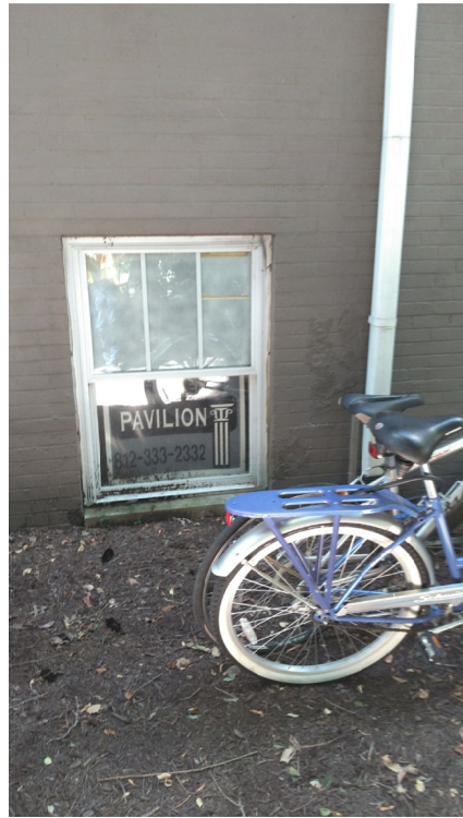
PROPOSED TELECOM MAKE BUILDING ENTRANCE INTO STORAGE AREA LINEAL LEAVE TAIL OF .75"TD AT BUILDING WALL FOR TELECOM
