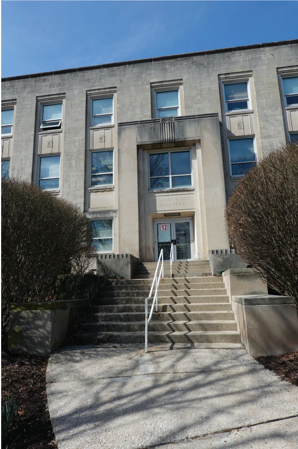
Photo 3. East Entry Detail
