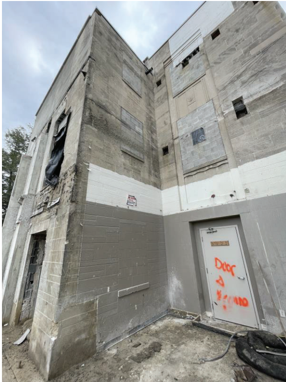
Photo 6. Northwest Corner of North Stair
