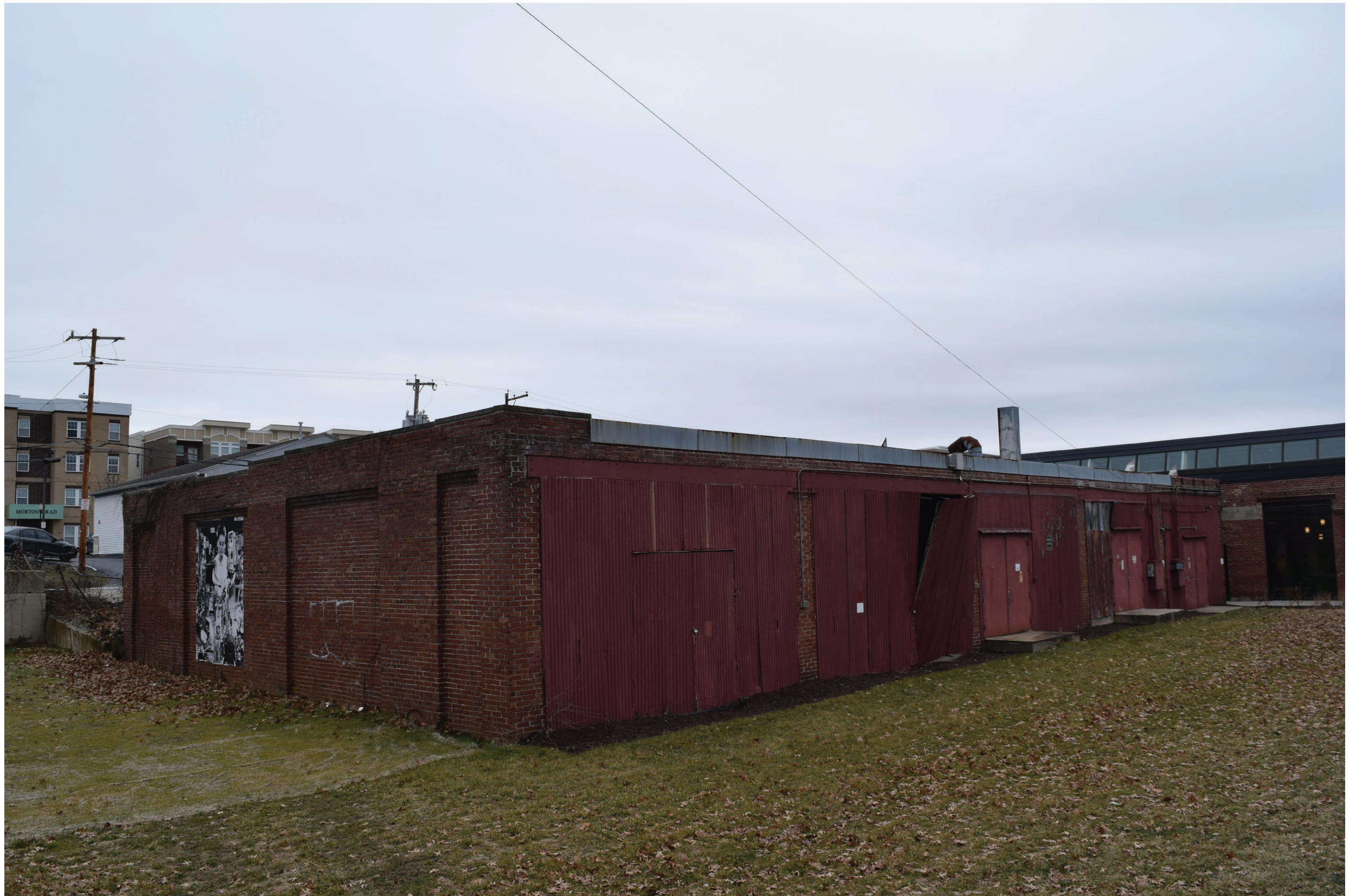
EXISTING KILN STRUCTURE
