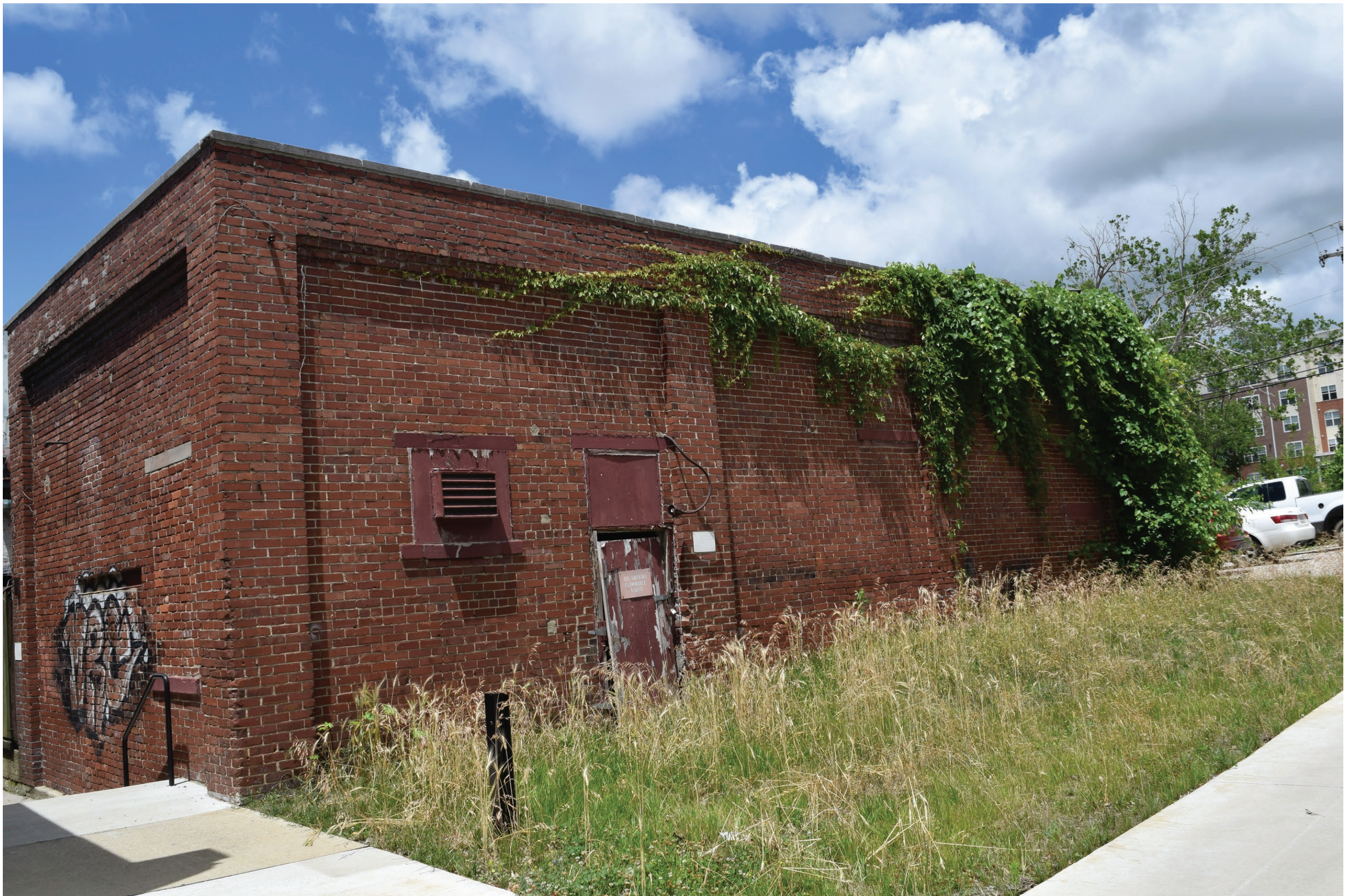
EXISTING POWER HOUSE STRUCTURE
