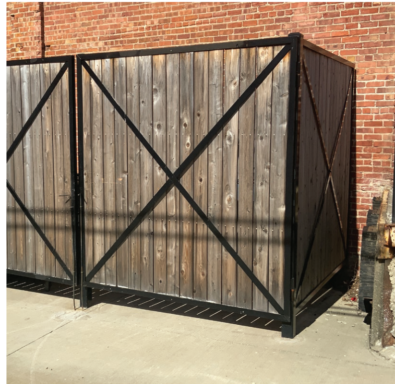
SILVERED CEDAR AND BLACK PAINTED STEEL AT THE MILL
