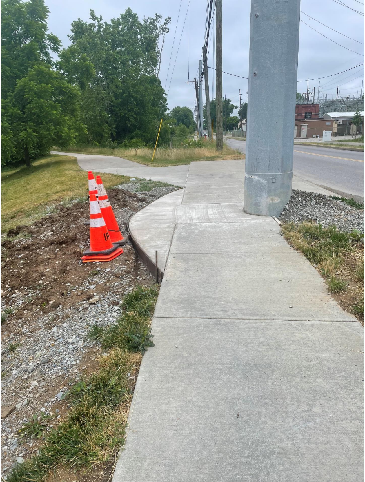
Photo 7 Sidewalk opened, facing south. June 12th, 2023
