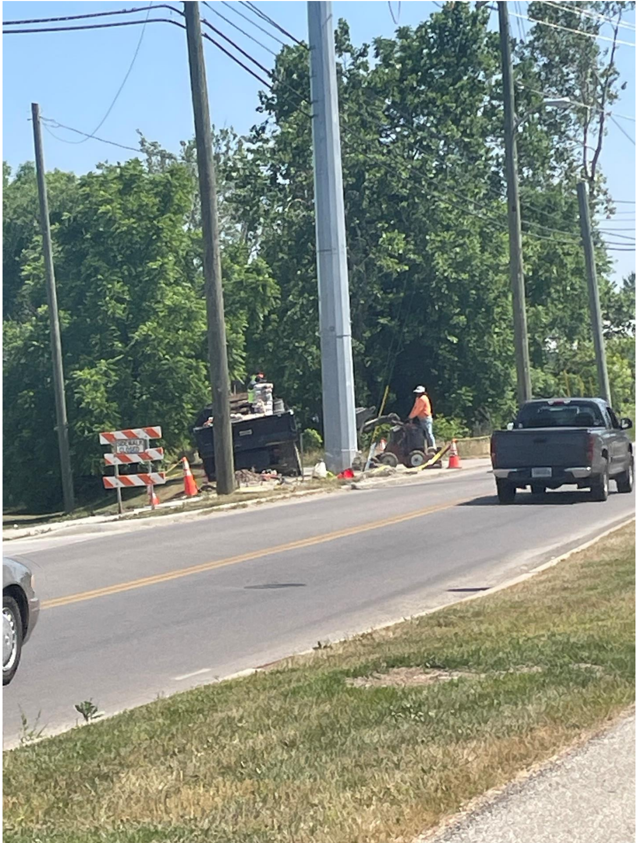
Photo 6 Work taking place at obstruction, facing southeast. June 9th, 2023
