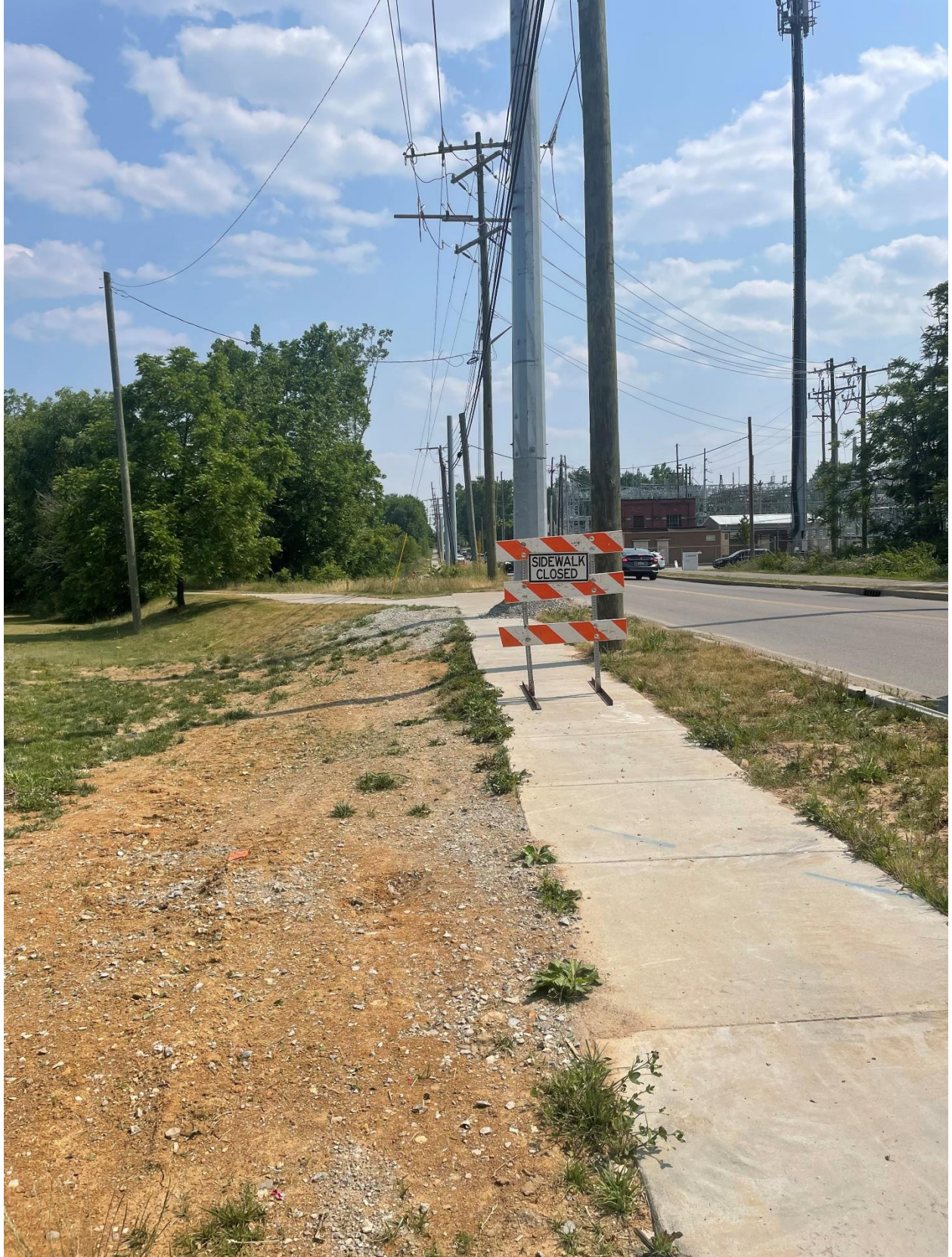
Photo 4 Barricade in place at obstruction, facing south. June 8th, 2023
