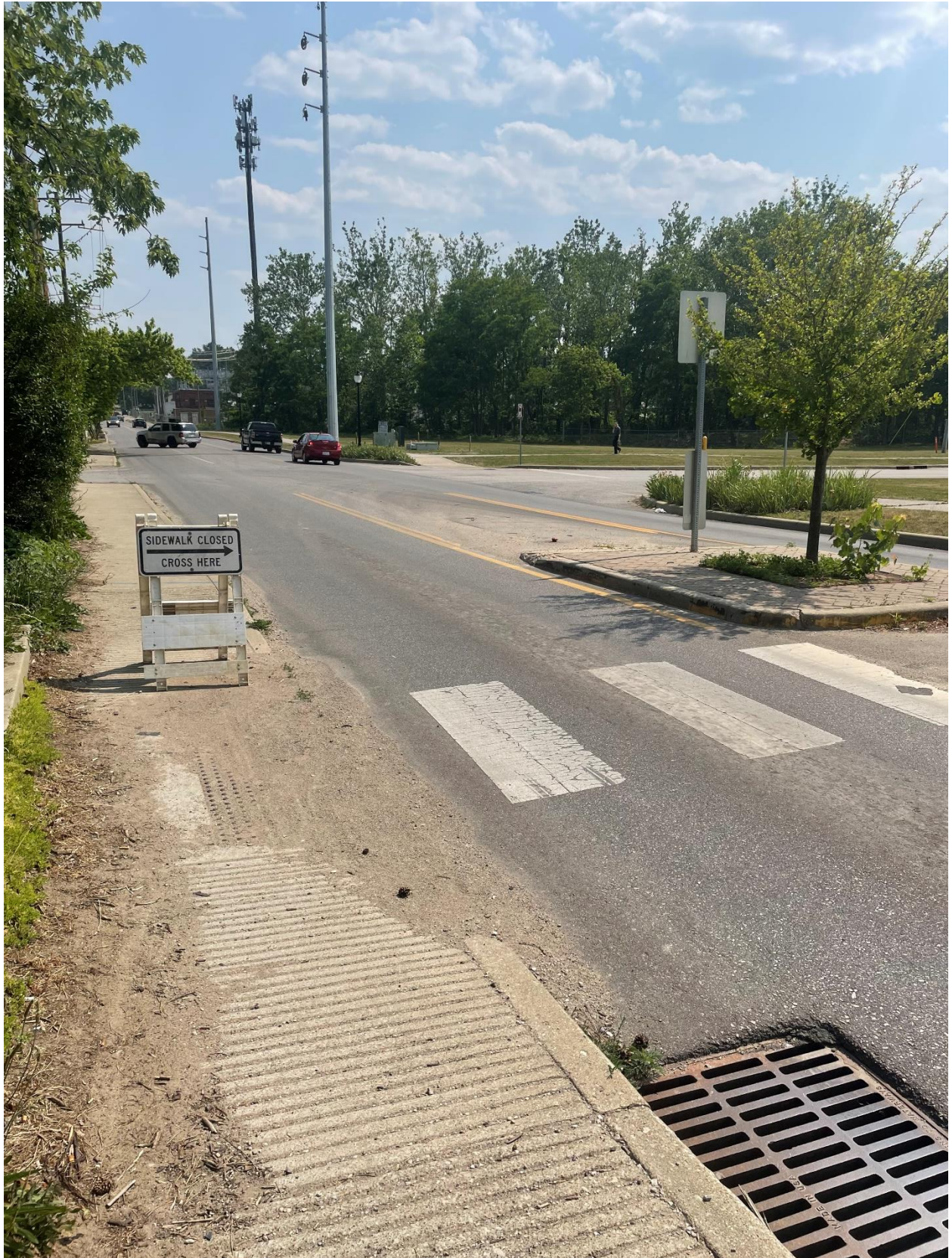
Photo 3 Advanced warning of sidewalk closure at crosswalk. North of obstruction, facing south. June 8th, 2023
