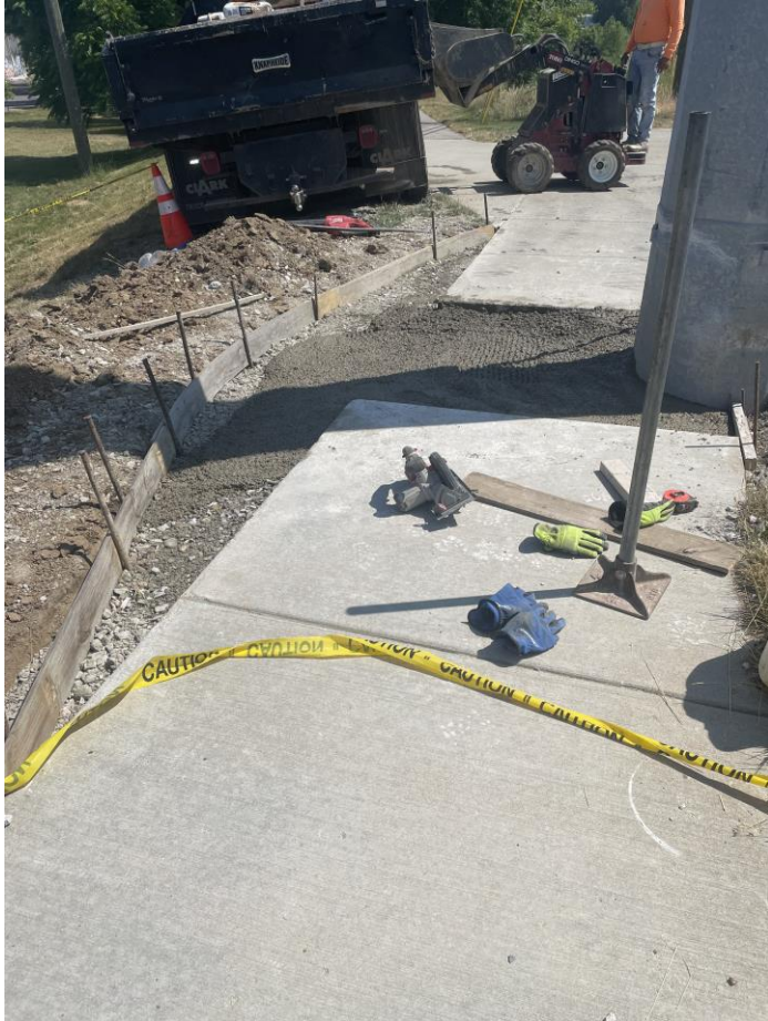
Photo 3: Sidewalk restoration with bag concrete mix 6/9/2023
