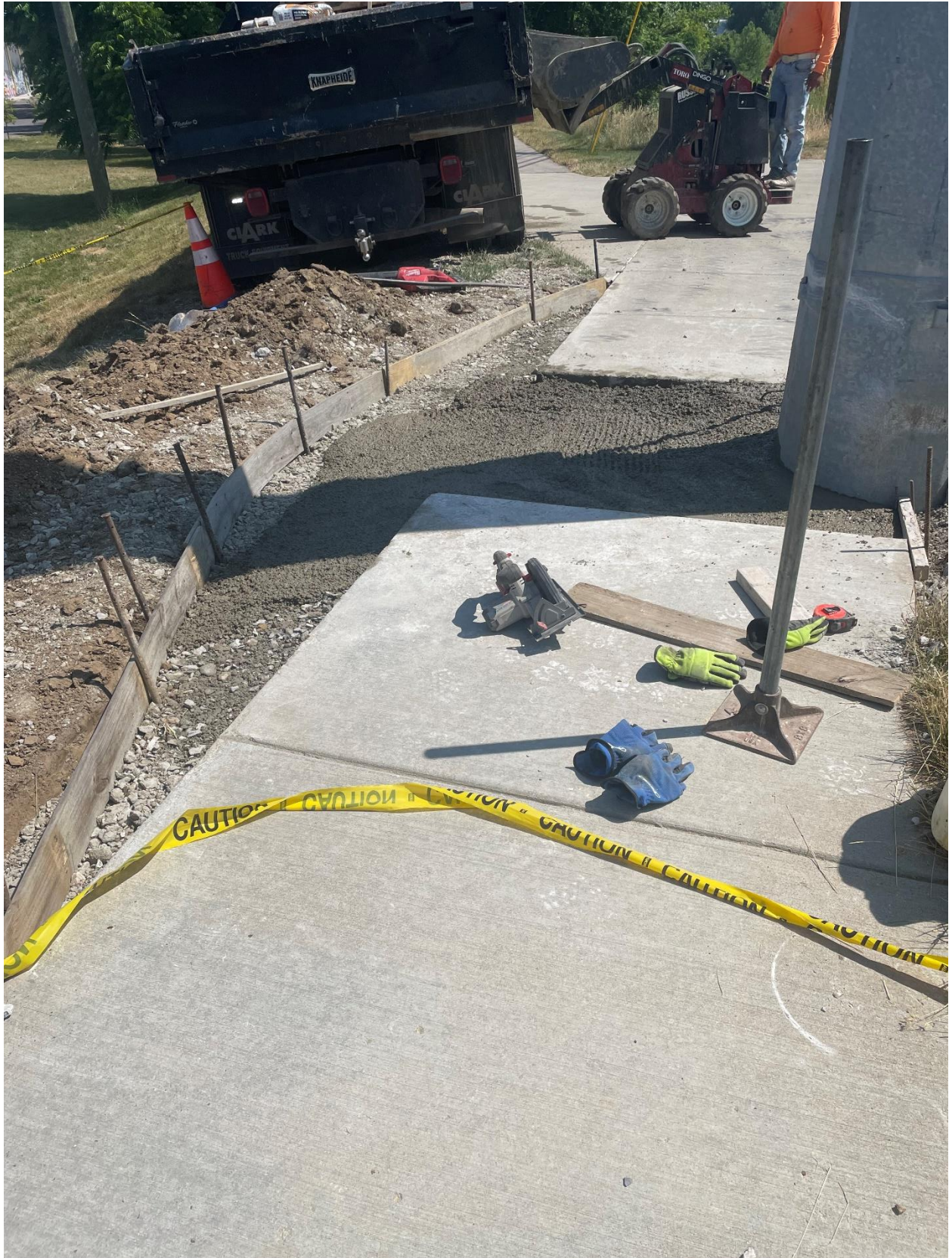
Photo 5 Work taking place at obstruction, facing south. June 9th, 2023
