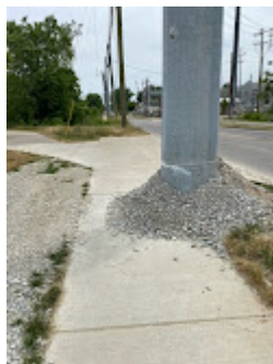
Pole at S Rogers - Warehouse.jpeg 153K
