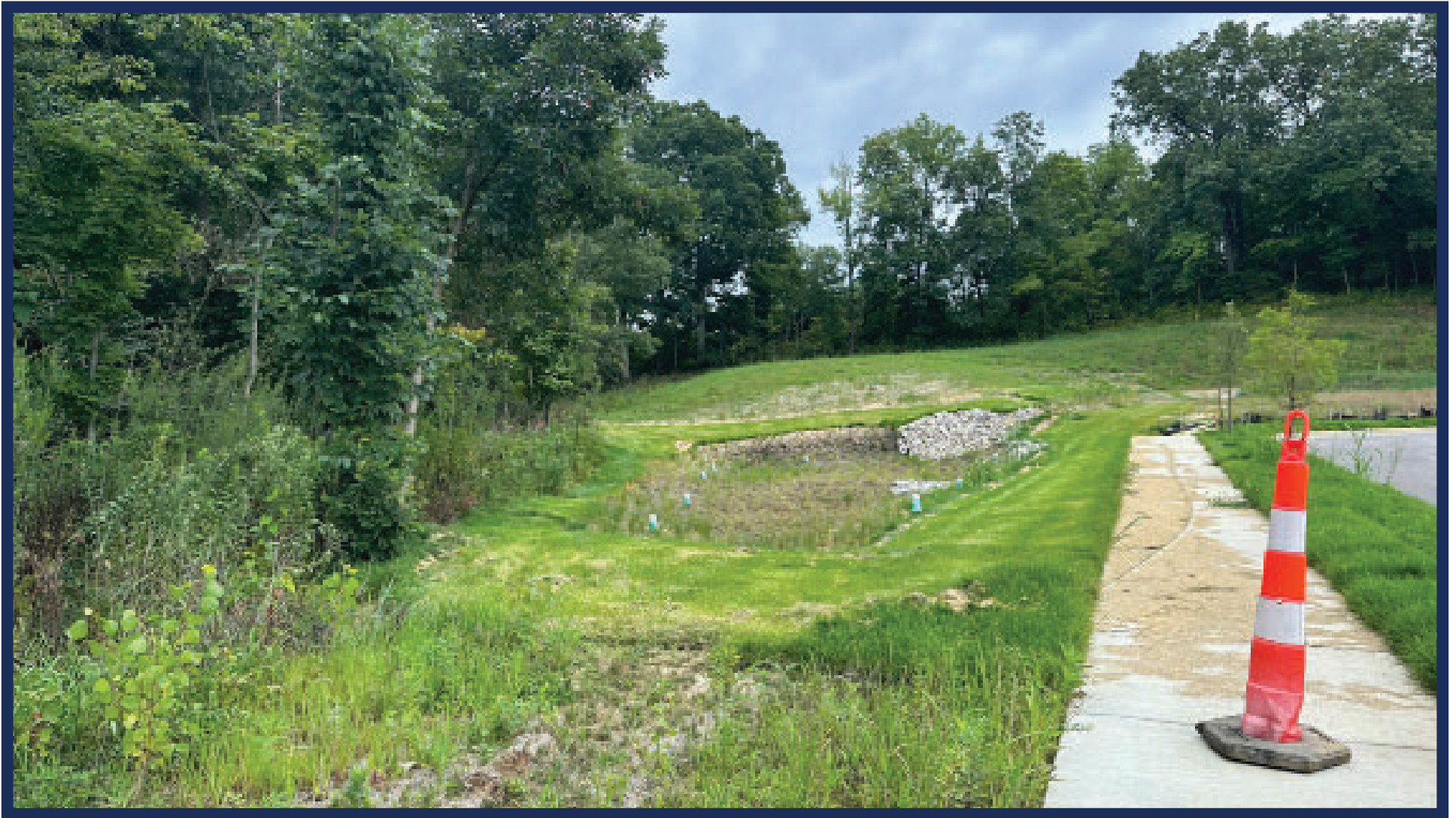
Arlington Park Photo 3 Site Visit August 15, 2023 View standing on the north and looking towards the north east
