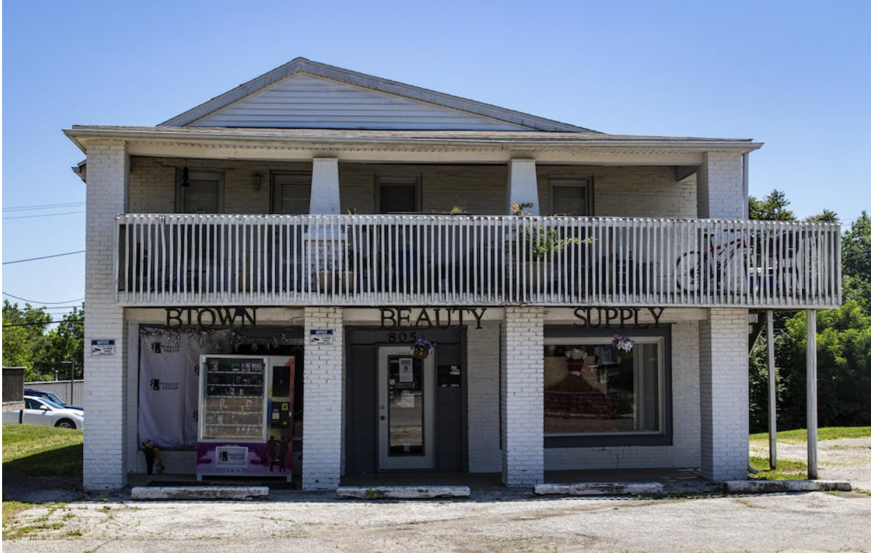
EXTERIOR OF BUILDING
