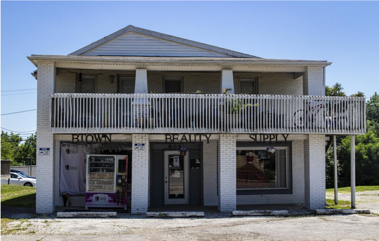
EXTERIOR OF BUILDING
