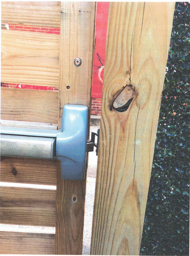
Current patio doors with large gap near latch.
