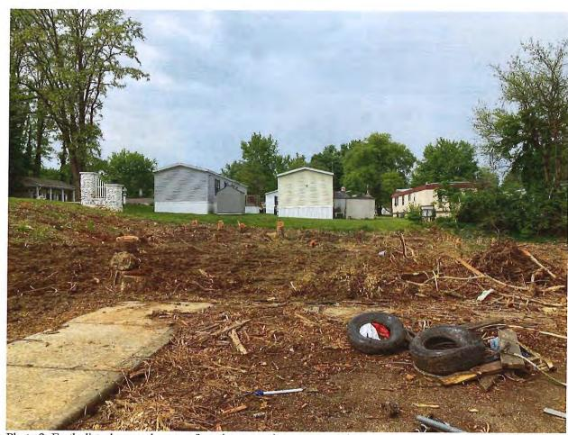
Photo 2: Earth disturbance, absence of erosion control measures, and trees removed on the northern side of 1450 N Willis Drive on 05/16/2023.
