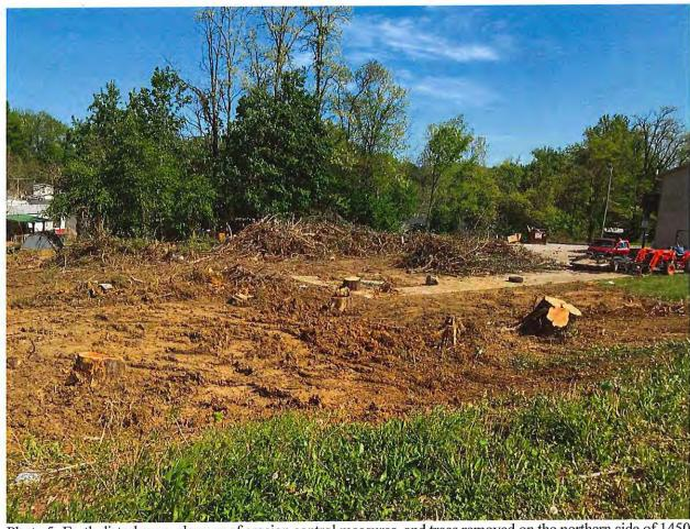
Photo 5: Earth disturbance, absence of erosion control measures, and trees removed on the northern side of 1450 N Willis Drive on 05/09/2023.
