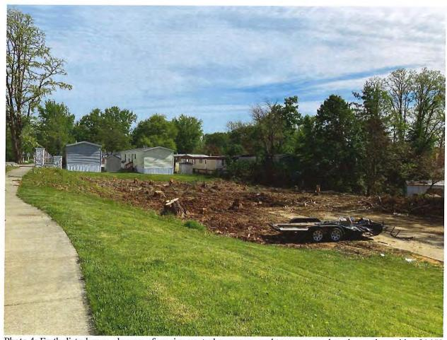
Photo 4: Earth disturbance, absence of erosion control measures, and trees removed on the northern side of 1450 N Willis Drive on 05/11/2023.
