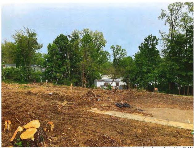
Photo 1: Earth disturbance, absence of erosion control measures, and trees removed on the northern side of 1450 N Willis Drive on 05/16/2023.
