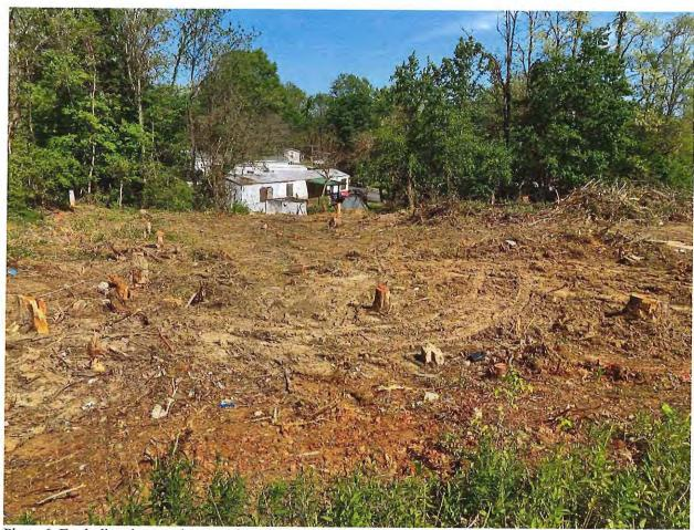
Photo 6: Earth disturbance, absence of erosion control measures, and trees removed on the northern side of 1450 N Willis Drive on 05/09/2023.
