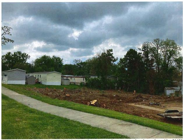
Photo 3: Earth disturbance, absence of erosion control measures, and trees removed on the northern side of 1450 N Willis Drive on 05/12/2023.
